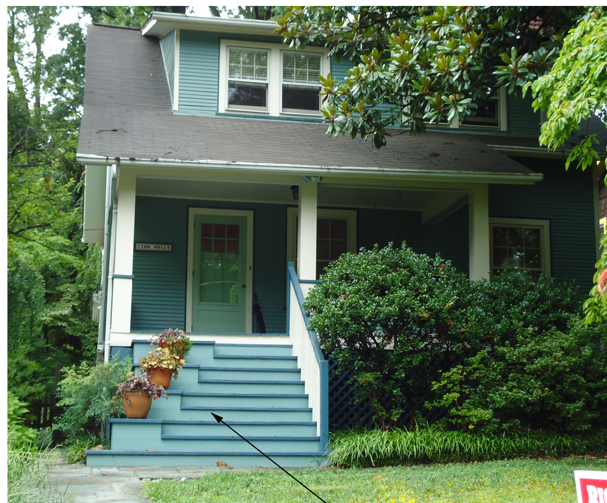
Front Porch Steps - current condition
