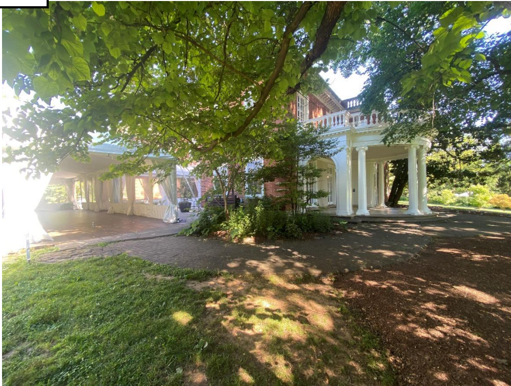
Woodend: East walkway from terrace to portico
