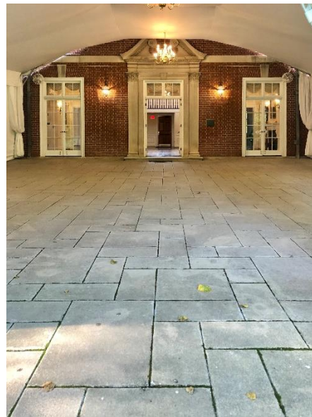
Existing Concrete Pavers
