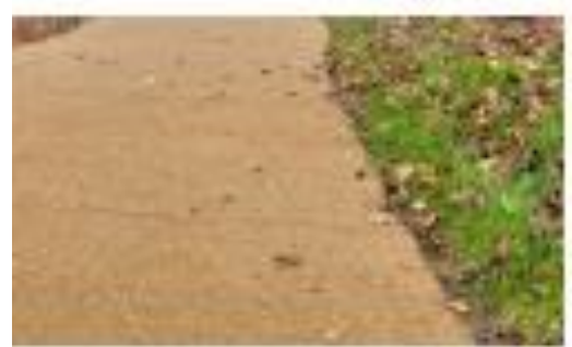
#3 – New material for path from terrace to portico is permeable stone flexipave, which was approved as a material in HAWP #35/12-19D.
