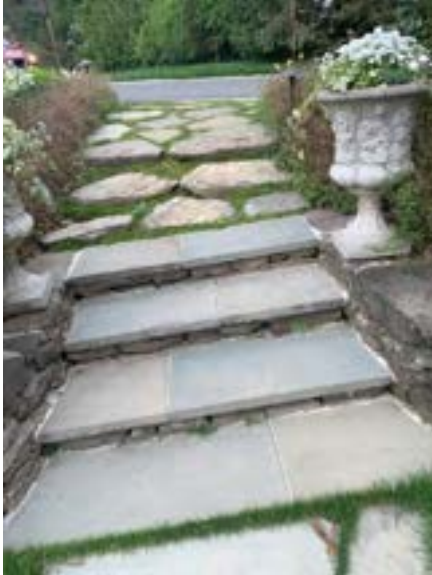
Steps at Patio – Flagstone Treads with Fieldstone Risers
