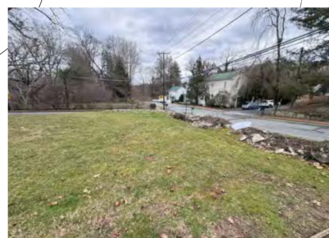
View of Existing Stone Wall to be Re-Stacked - Wall width to be between 24" to 30"
