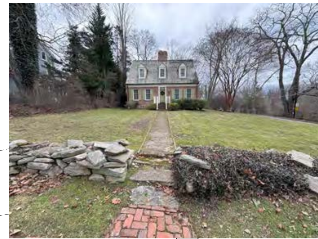
Existing Retaining Wall to be Re-stacked. View of Ex. Lead Walk to be Reset. Existing Stones to remain, but possibly Reset - TBD on site w/ Mason
