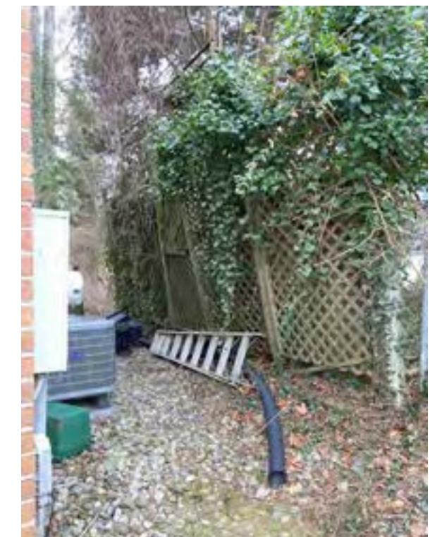
Existing Lattice Screen to be Removed
