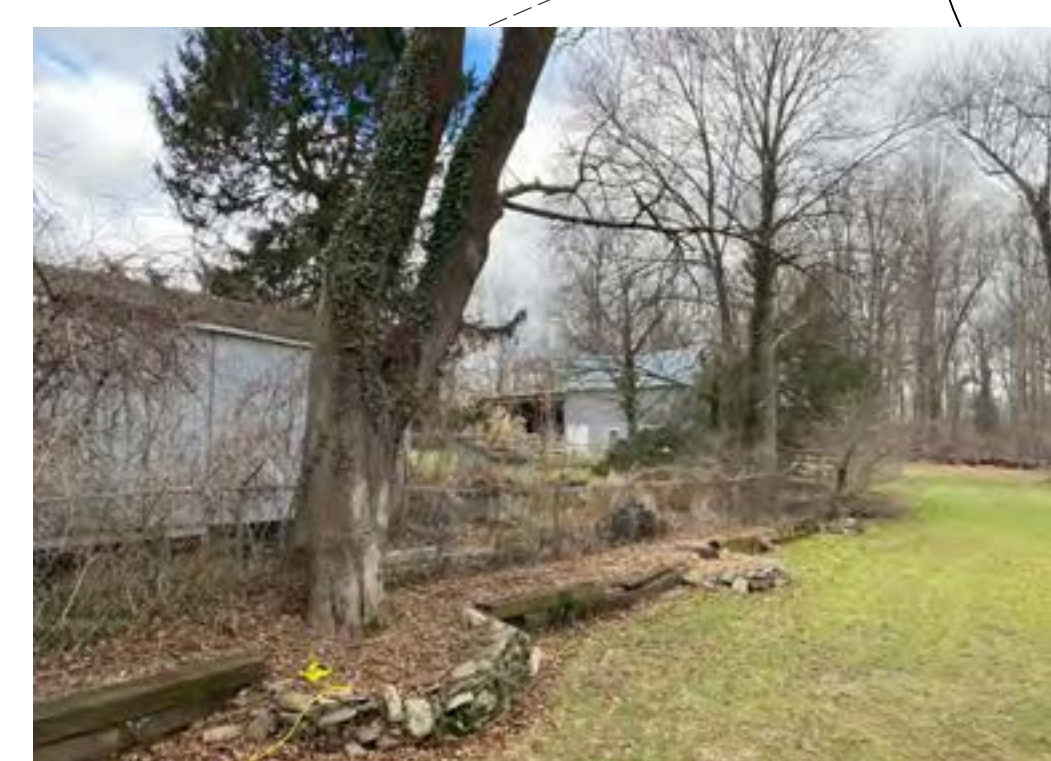
View of Existing Timber Retaining Wall to be Replaced Existing Stone wall to be removed + Feather out the Grade
