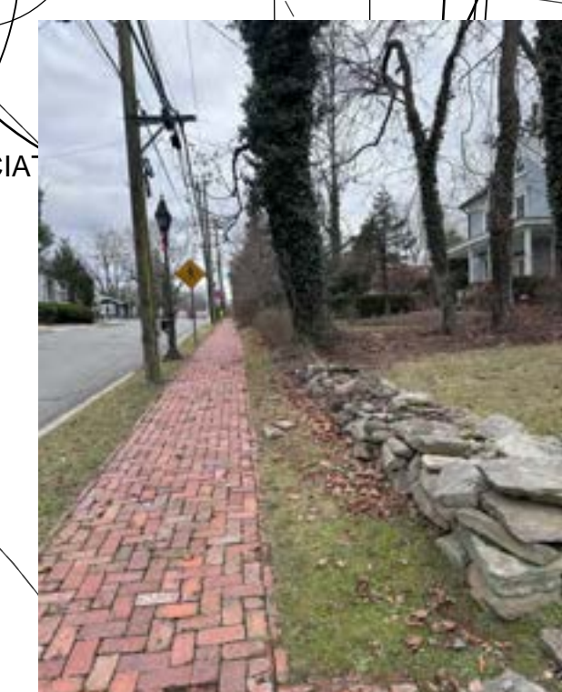
Existing Retaining Stone Wall and Public Side Walk
