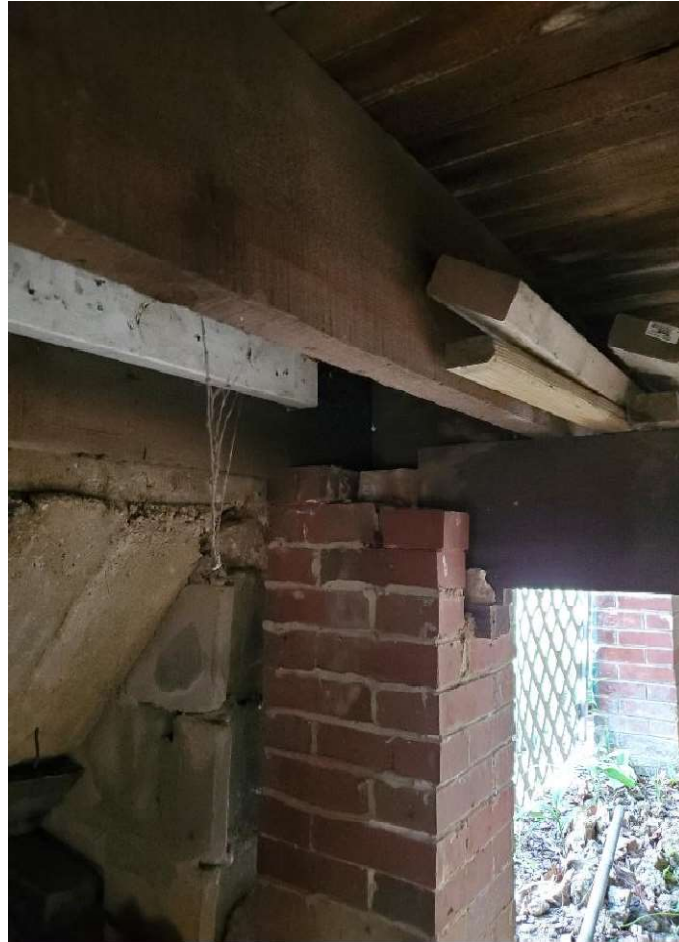
Photo 18 - 7102 Maple Ave – brick pier
