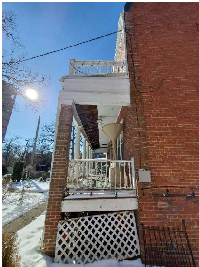
Photo B - 7102 Maple Ave – Side Elevation-North
