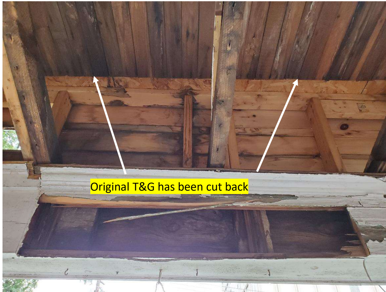
Photo 16 - 7102 Maple Ave – ‘wall’ above support beam
