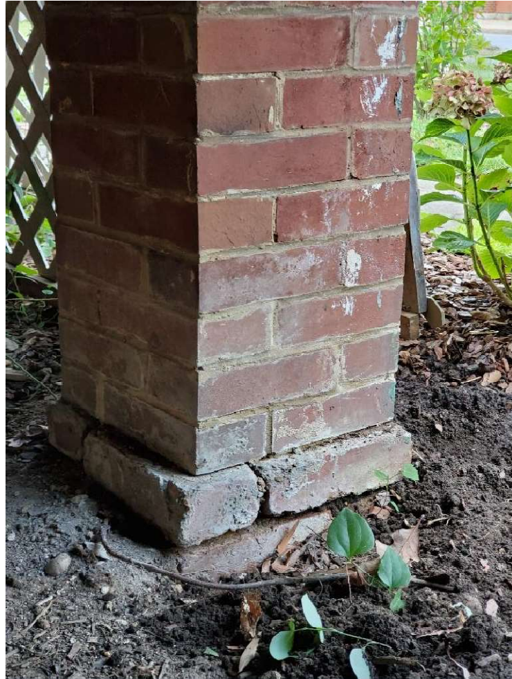
Photo 13 - 7102 Maple Ave – brick pier base
