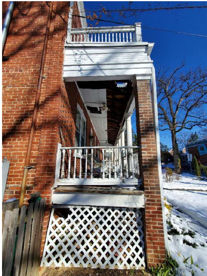
Photo C - 7102 Maple Ave – Side Elevation-South
