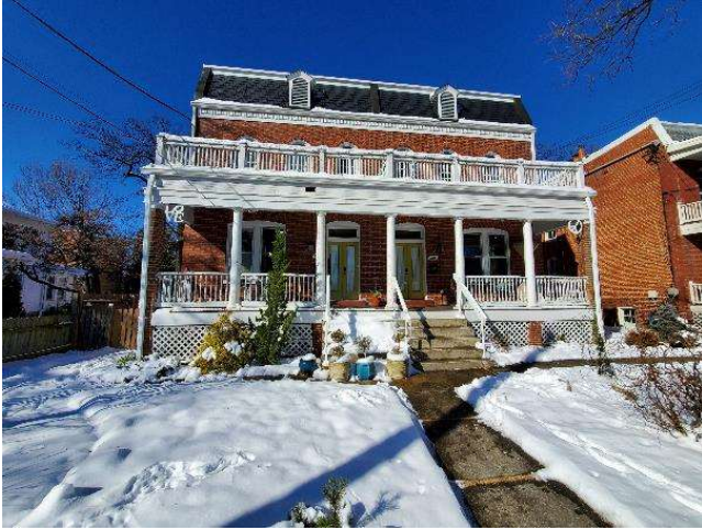
7102-4 Maple Ave – Fascia
