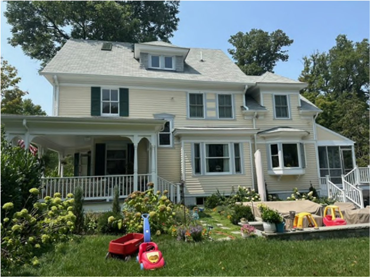
East façade – view 2.
