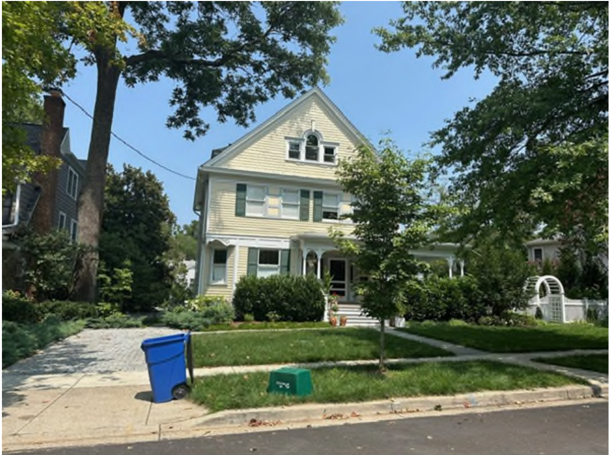
South View with downward sloping side yard shown.
