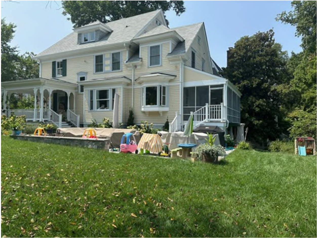
East Façade – view 1.
