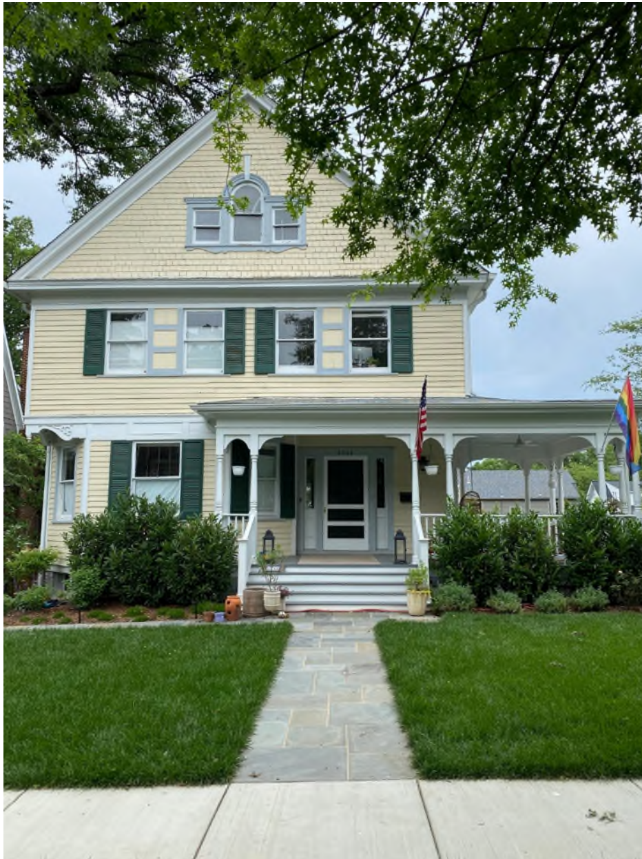
South View – Close Up of Front Facade
