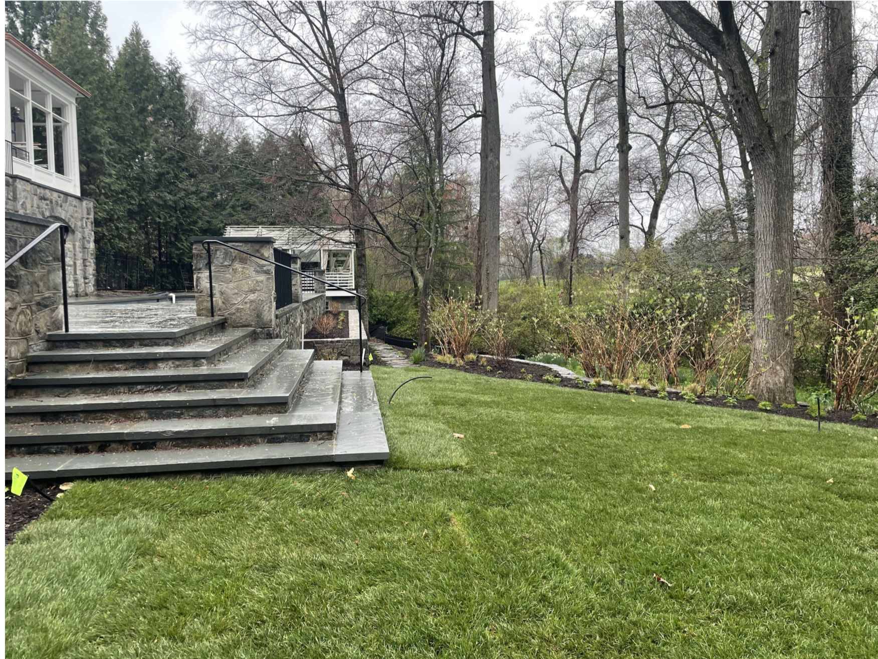
EXISTING STAIRS TO LOWER LAWN
