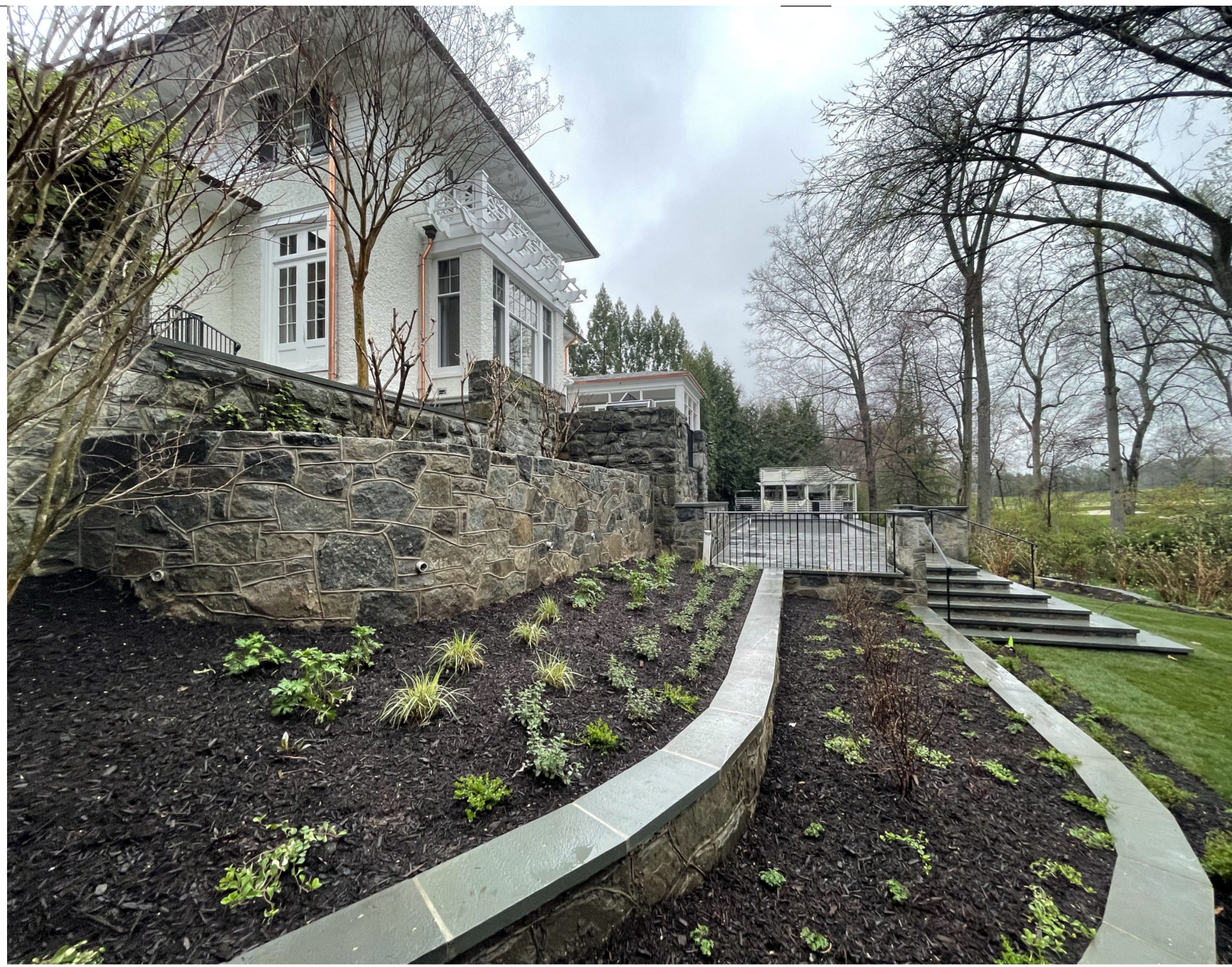
EXISTING TERRACE WALLS FROM REAR LAWN
