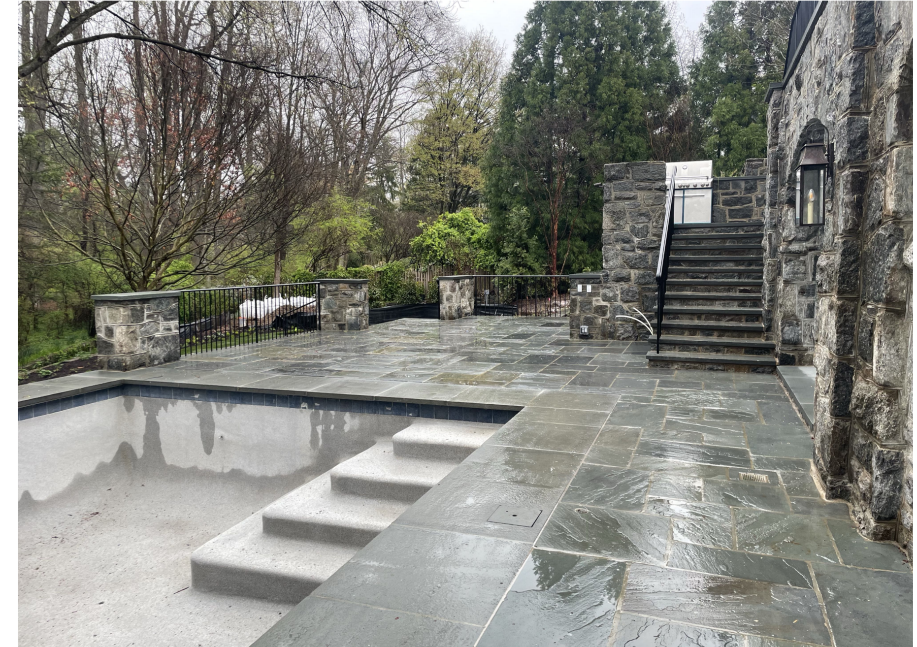
EXISTING POOL TERRACE AND STAIRS TO UPPER TERRACE
