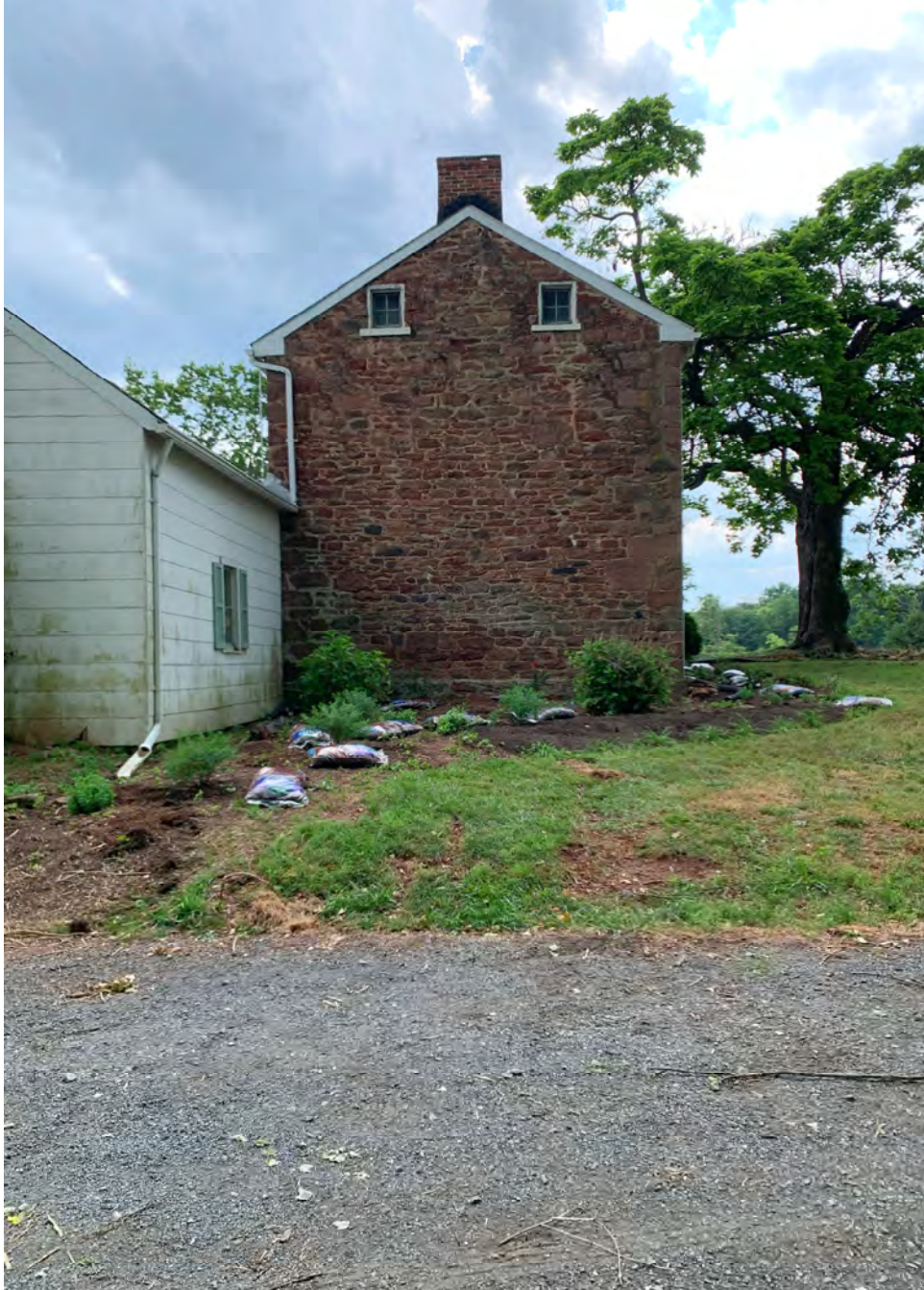
Valhala 1835 Stone House East View 2024
