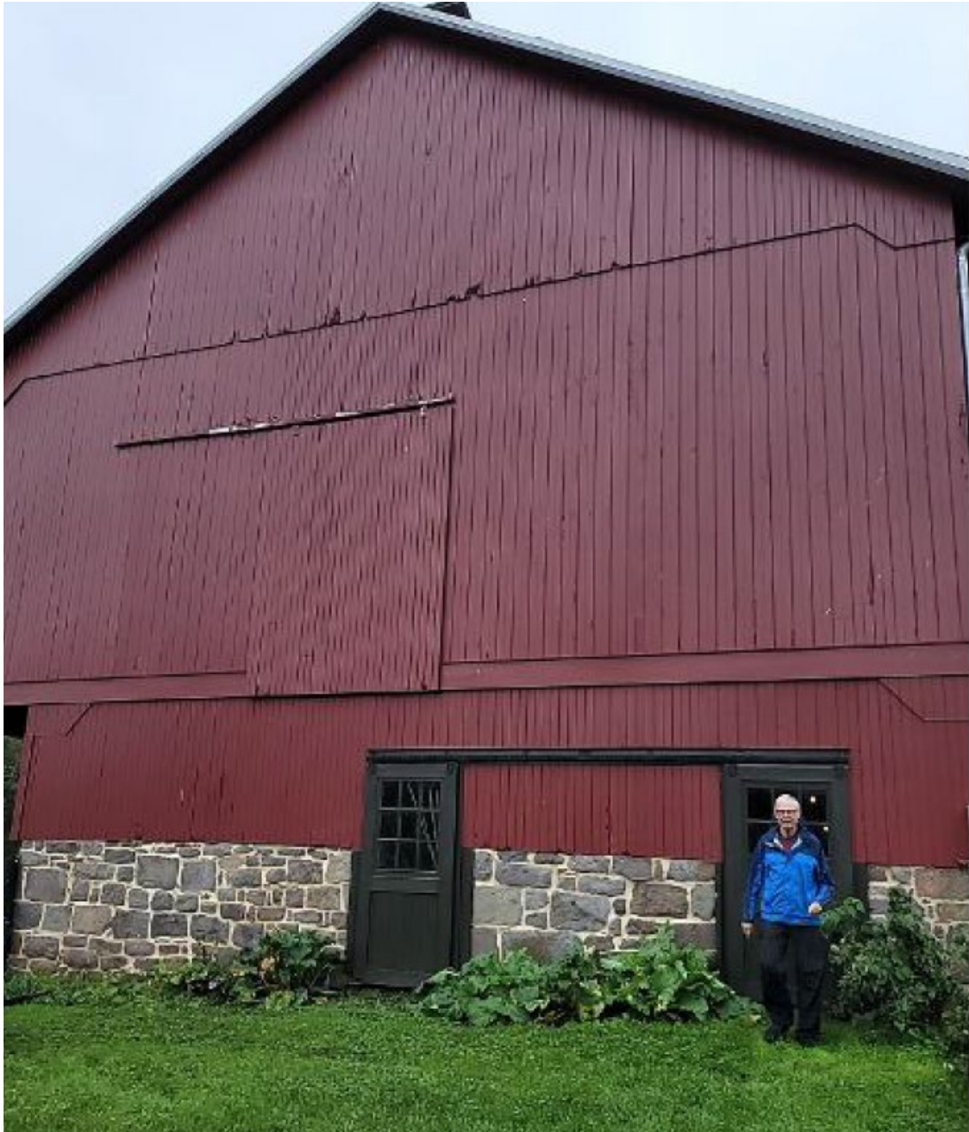
Front of Structure
