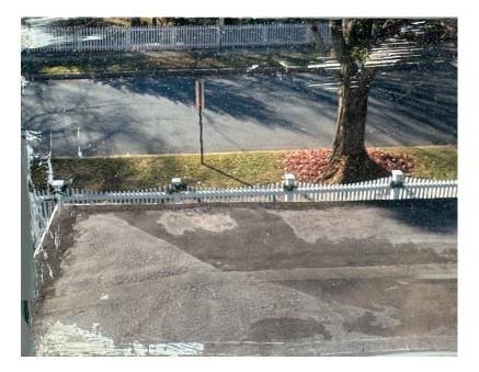
2. Current roof of the addition, taken from atop the main roof. Currently cracked with visible seams
