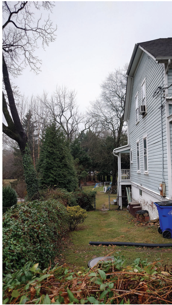
Left Side Photo Property line is in hedgerow
