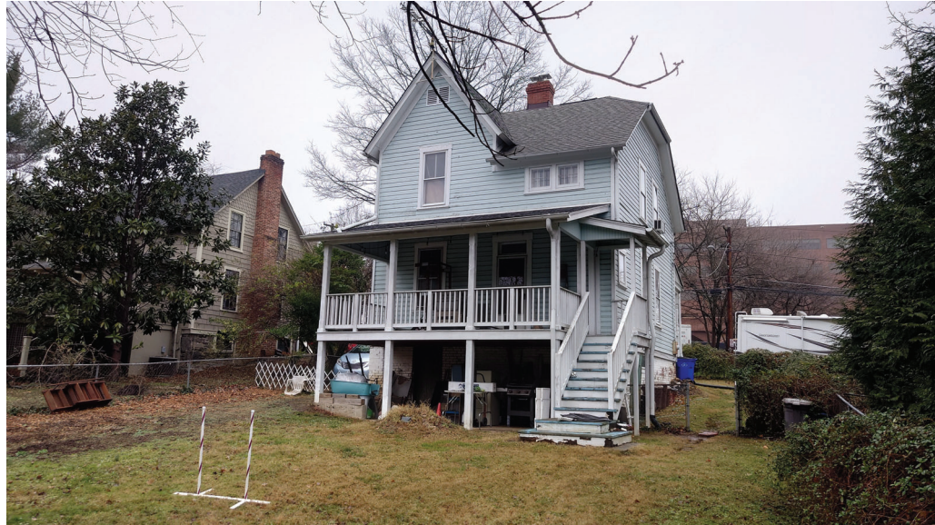
Rear Photo Wood porch to be removed
