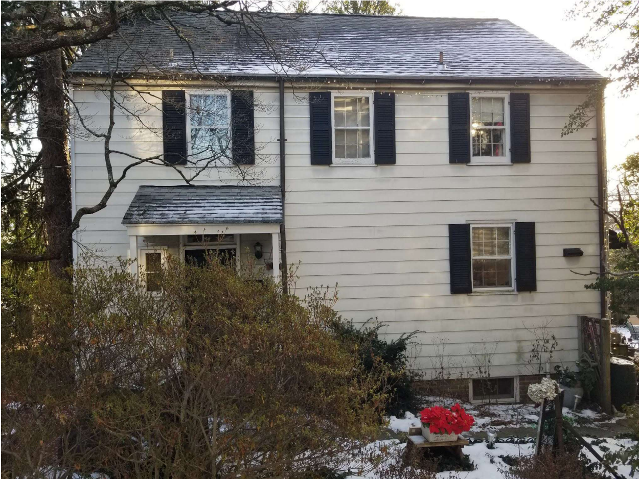
Gutter and downspouts on front (east side) of house
