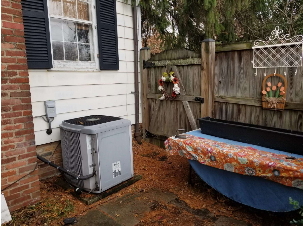
Downspout on NE corner of house
