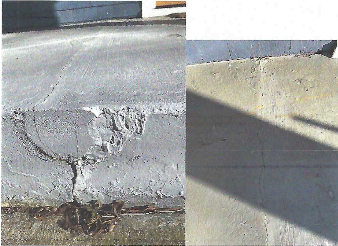
Cracks in the concrete slab and evidence of past repairs.
