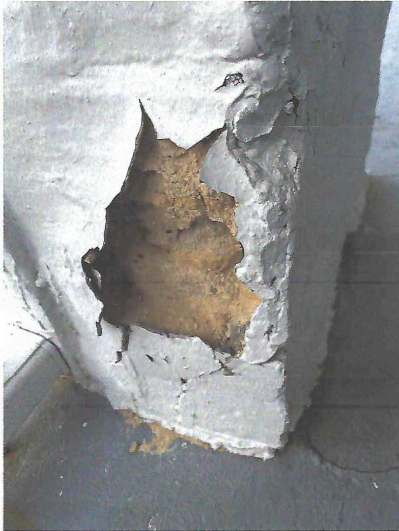
Deteriorating Brick. This is 5"W x 6"H
