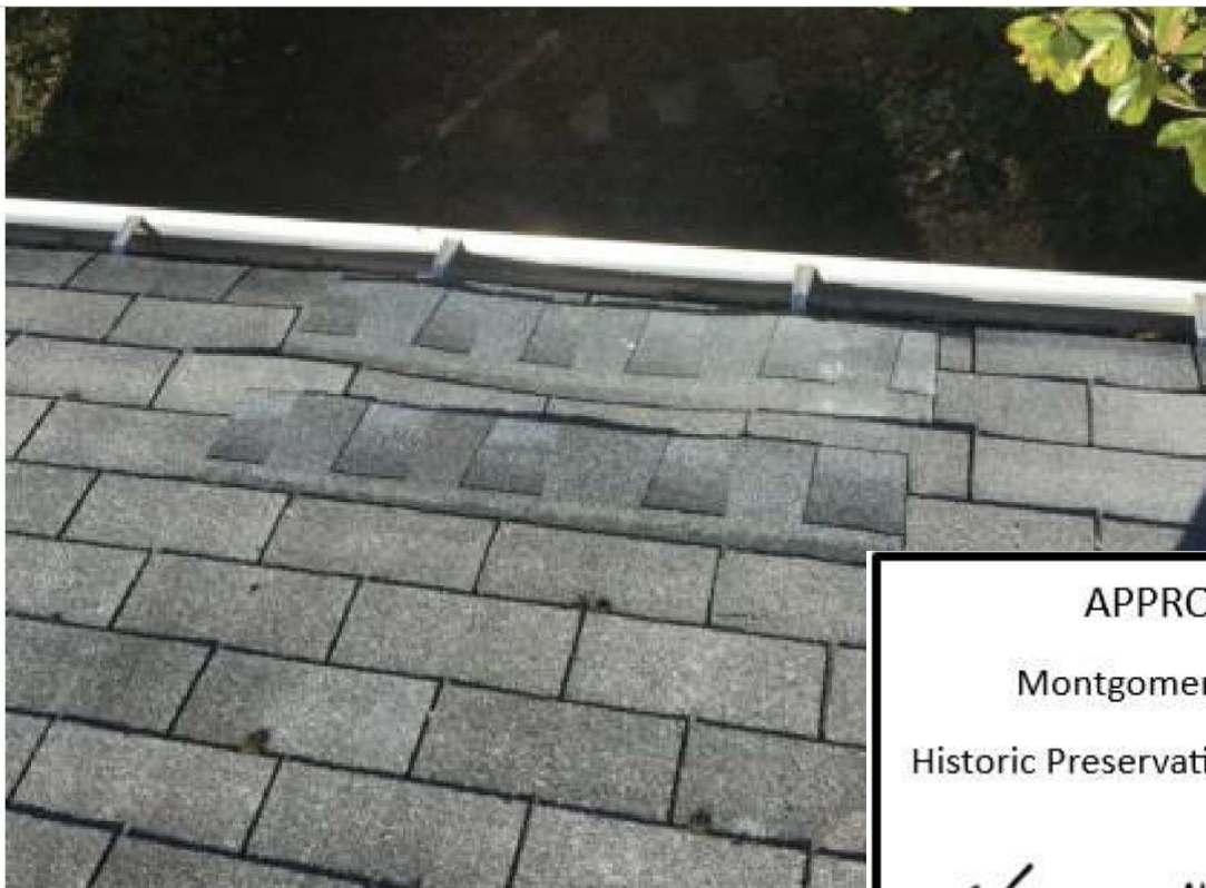
Sub-standard repairs made to old roof where leaking had occurred (atop old shingles)
