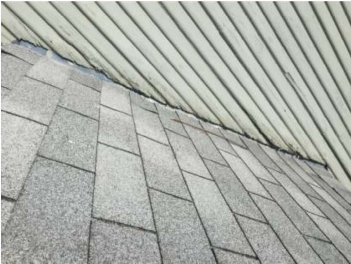
Shingles and failing flashing at Maple Ave. end of sun porch roof
