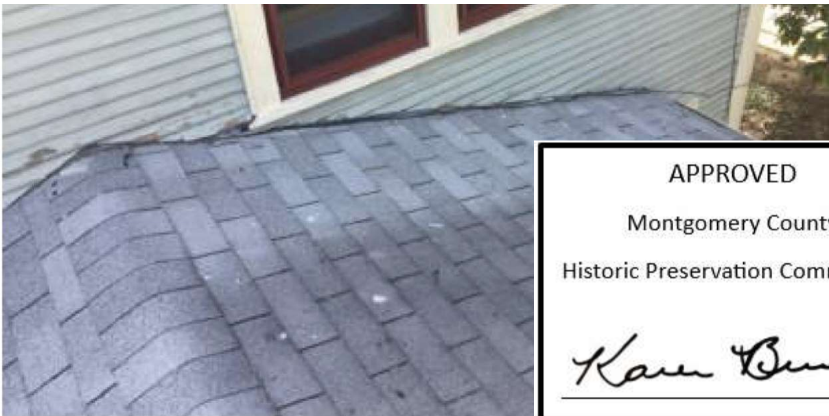
Shingles and failing flashing at Maple Ave. end of sun porch
