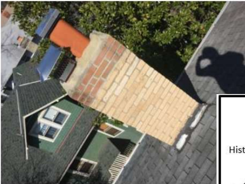
Poorly installed flashing at chimney
