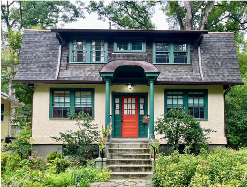
FRONT OF HOUSE: 8 DOUBLE-HUNG WINDOWS, 2 CASEMENTS
