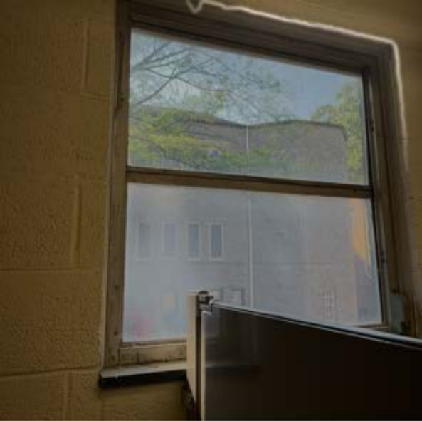
Photo 8: jalousie window inside restroom.
