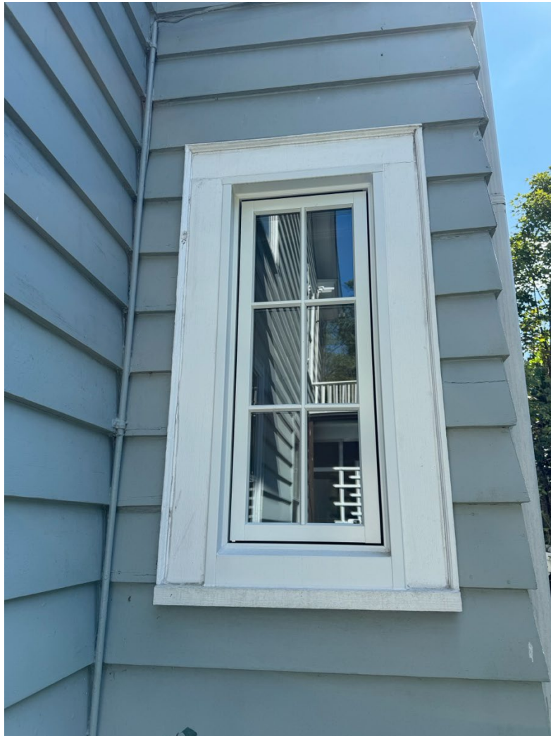
North Elevation first floor window (close up)
