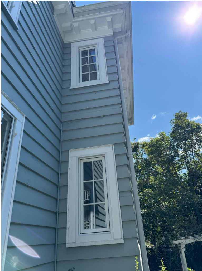
North Elevation first and second floor windows
