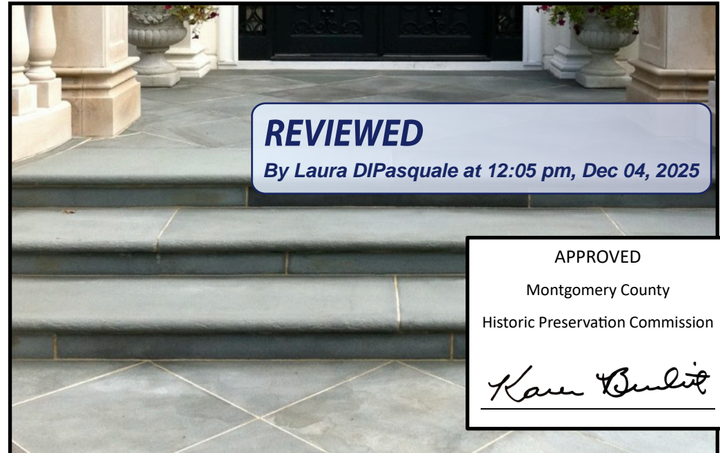
FRONT ENTRANCE WALK - THERMAL BLUE SELECT WITH BLUESTONE BORDER DIAMOND PATTERN PAVING
