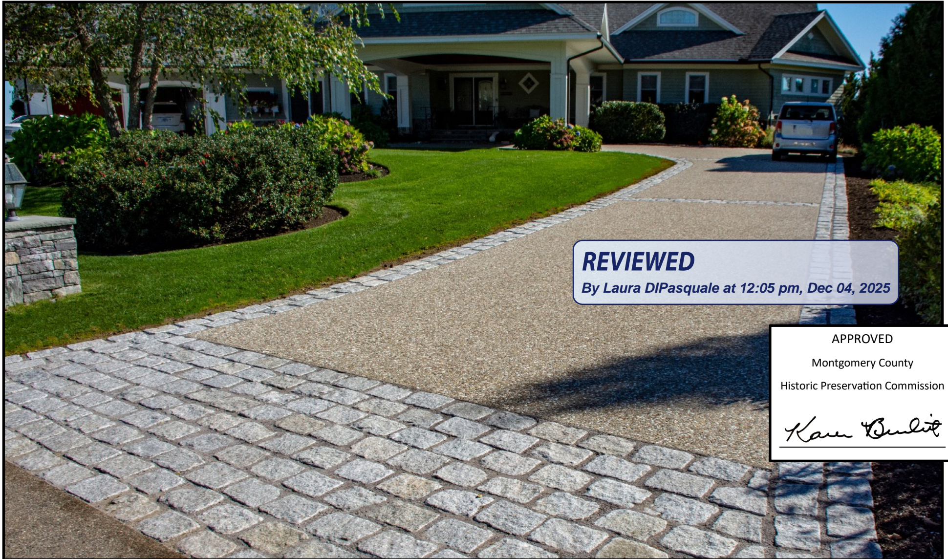
EXPOSED AGGREGATE WITH COBBLESTONE BORDER
