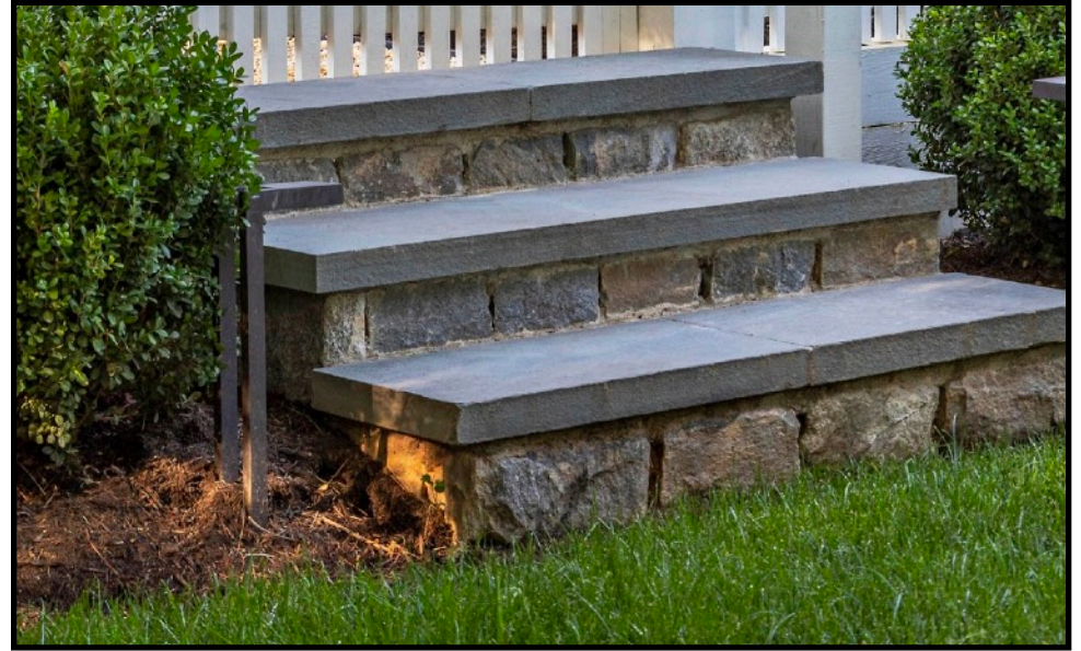
FRONT STEPS - STONE RISERS WITH THERMAL BLUESTONE STEPS
