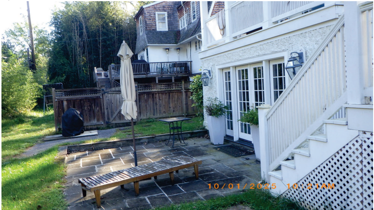
Figure 3. Existing stone patio and stairs to be removed to expand covered porch to proposed screened porch.
