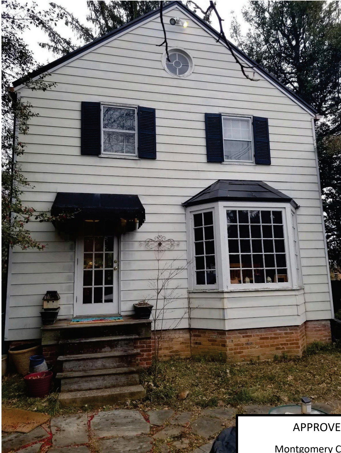
South side of the house showing rear entry, porch and steps
