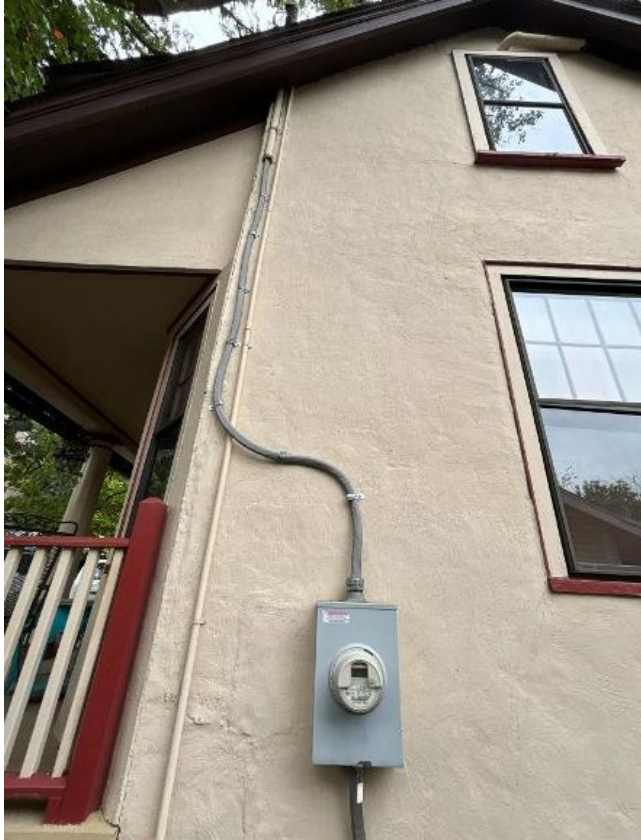
Utility Meter before Install
