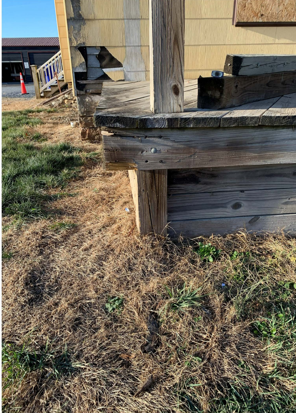
Holland House - Front Porch Deck Detail - December 2025
