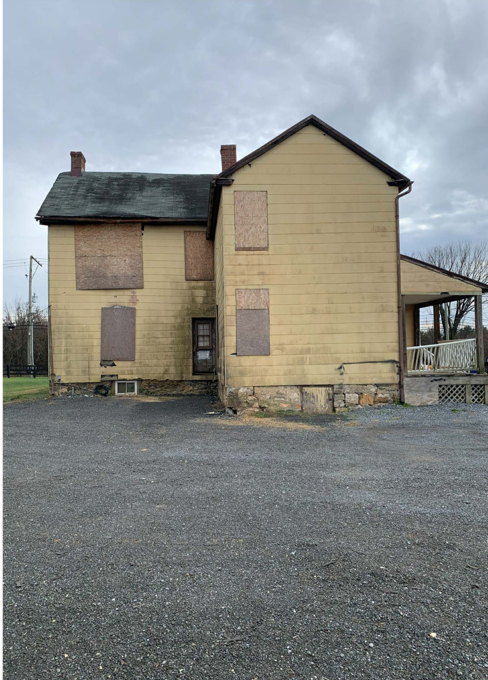
Holland House North Elevation - December 2025
