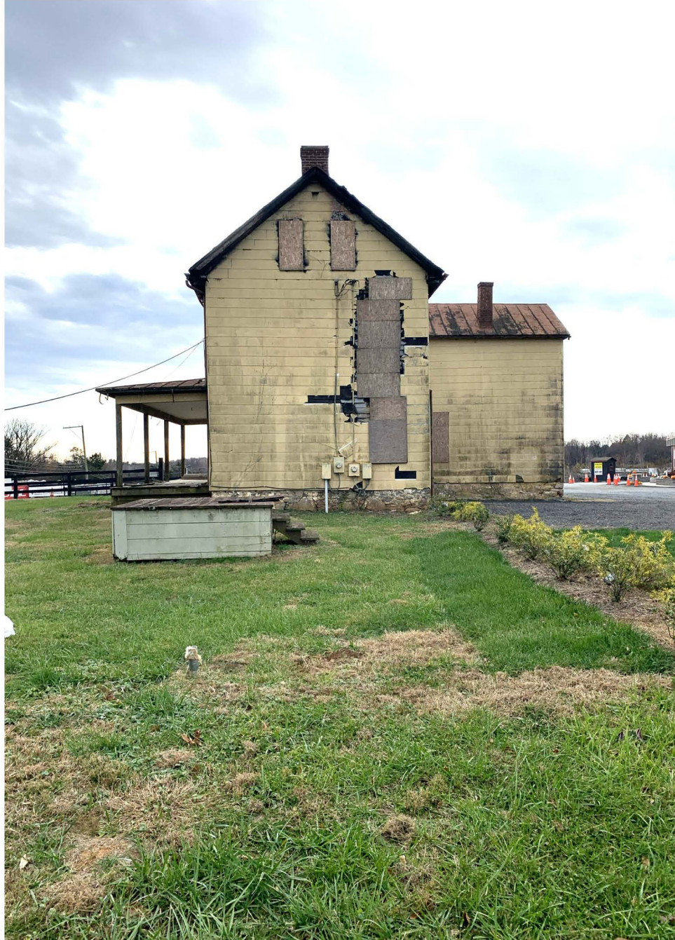
Holland House East Elevation - December 2025
