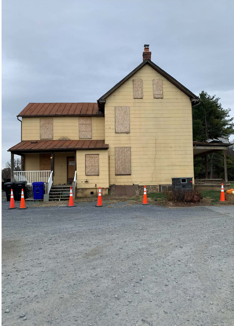
Holland House West Elevation - December 2025
