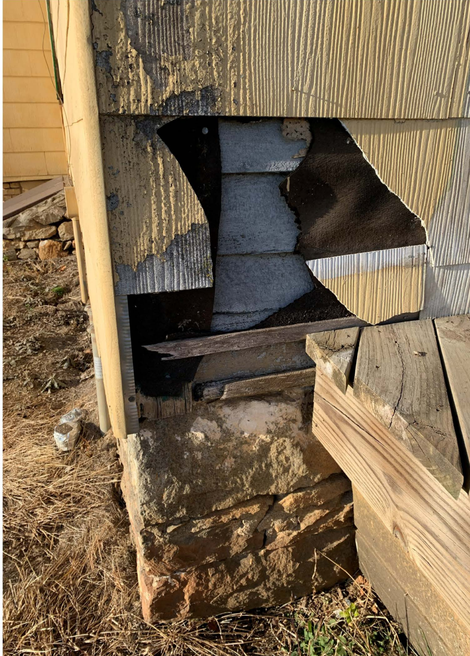
Holland House - Siding Detail at Southwest Corner - December 2025
