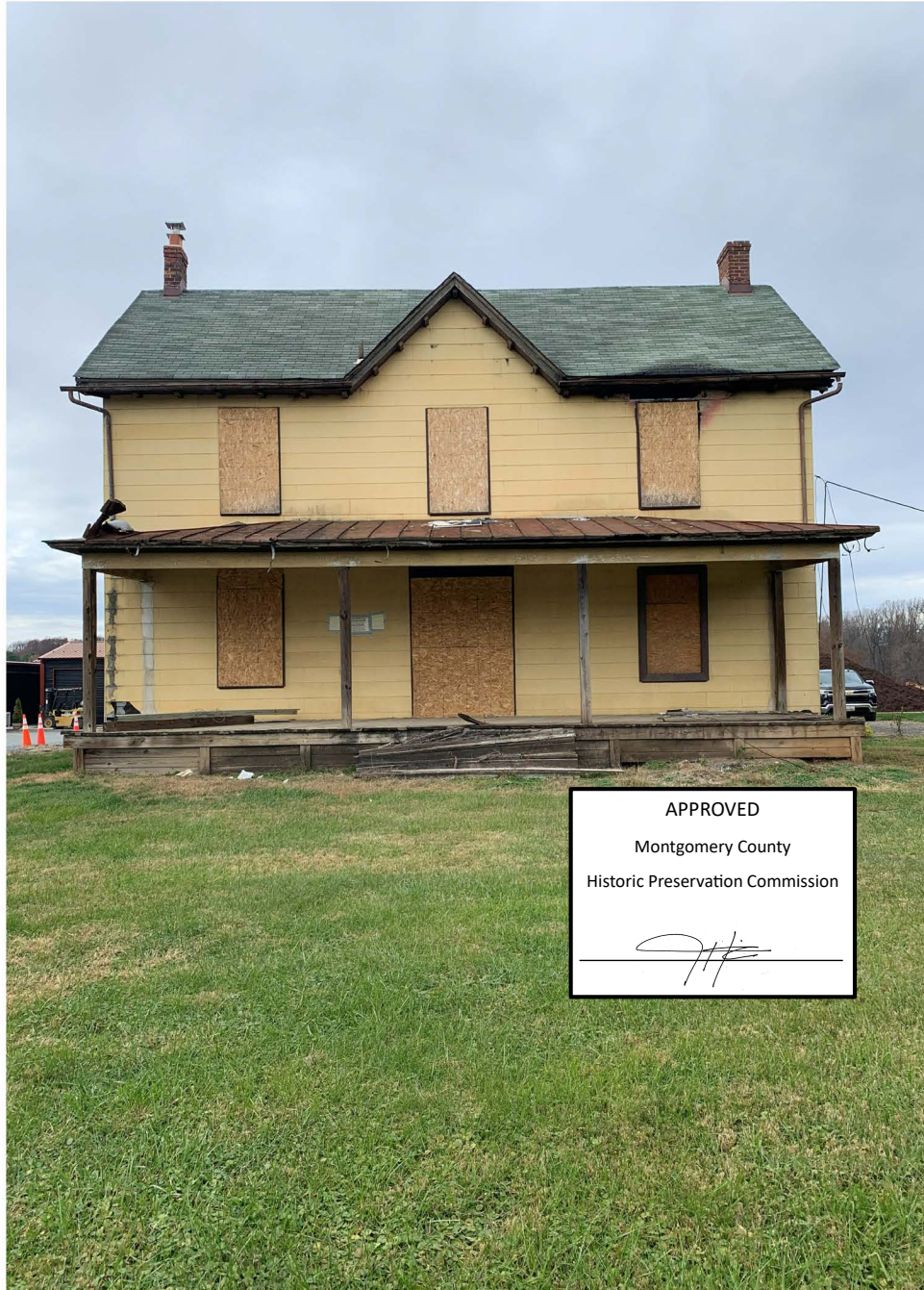
Holland House South Elevation - December 2025
