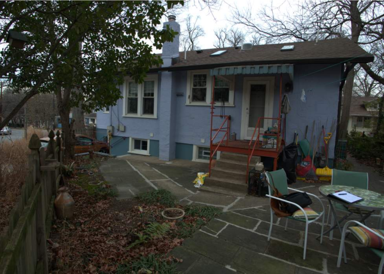
EXISTING REAR STAIRCASE & SLATE PATIO
