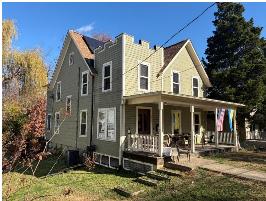
Figure 2 - House View from South (Takoma Avenue)
