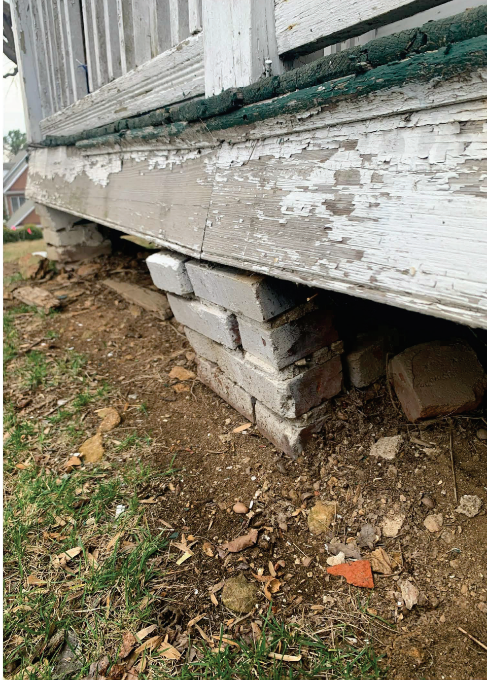
BMH Parsonage Brick Pier & Porch Framing at East Elevation - March 2026
