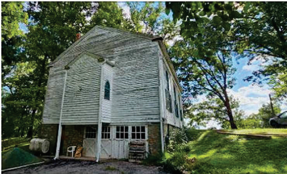
Bethesda Meeting House West Elevation View May 2025
