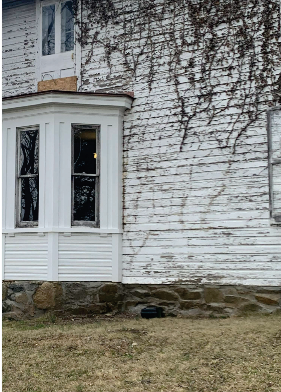
BMH Parsonage South Elevation Foundation- March 2026
