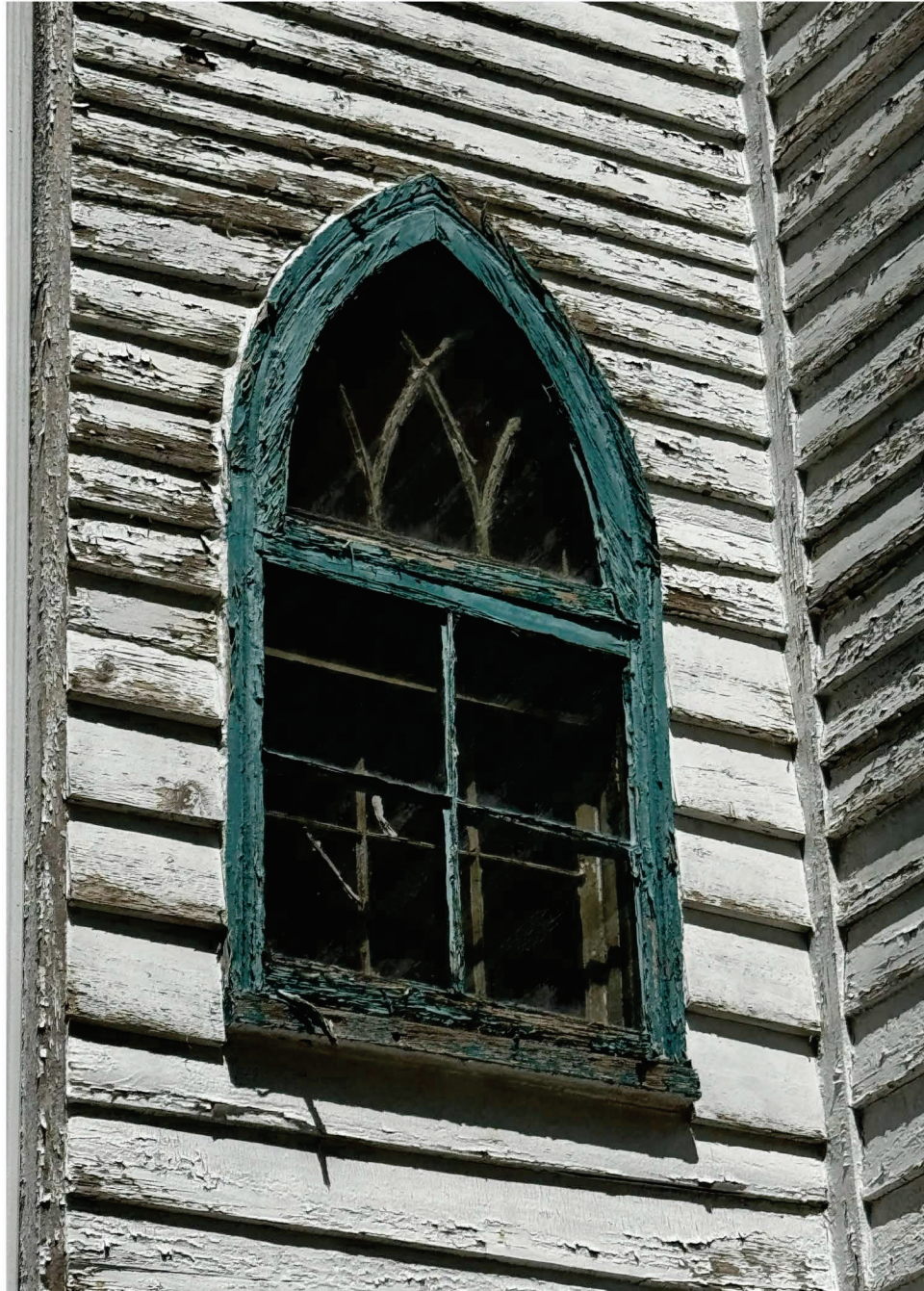
Bethesda Meeting House South Elevation Window at Alter April 2026
