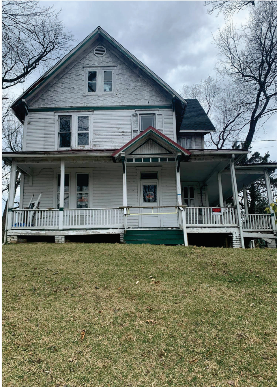
BMH Parsonage East Elevation - March 2026
