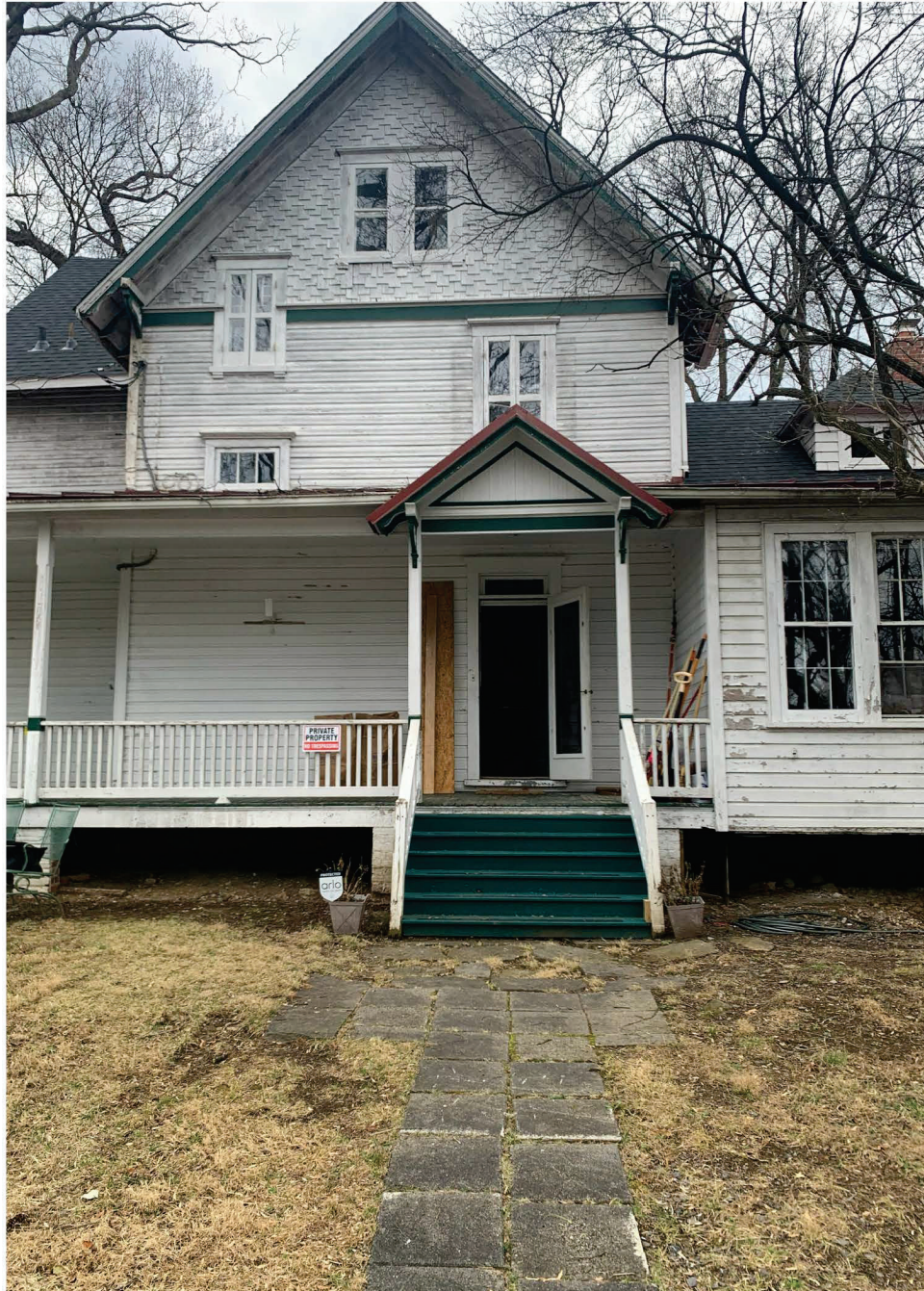
BMH Parsonage North Elevation - March 2026
