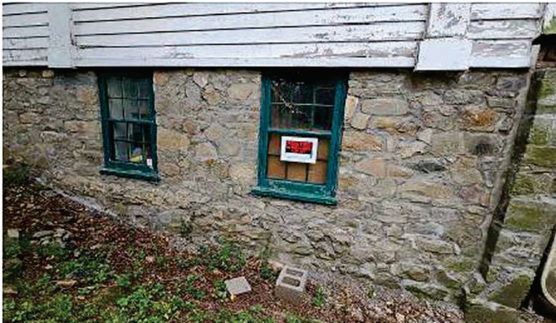
Bethesda Meeting House North Elevation View Foundation May 2025
