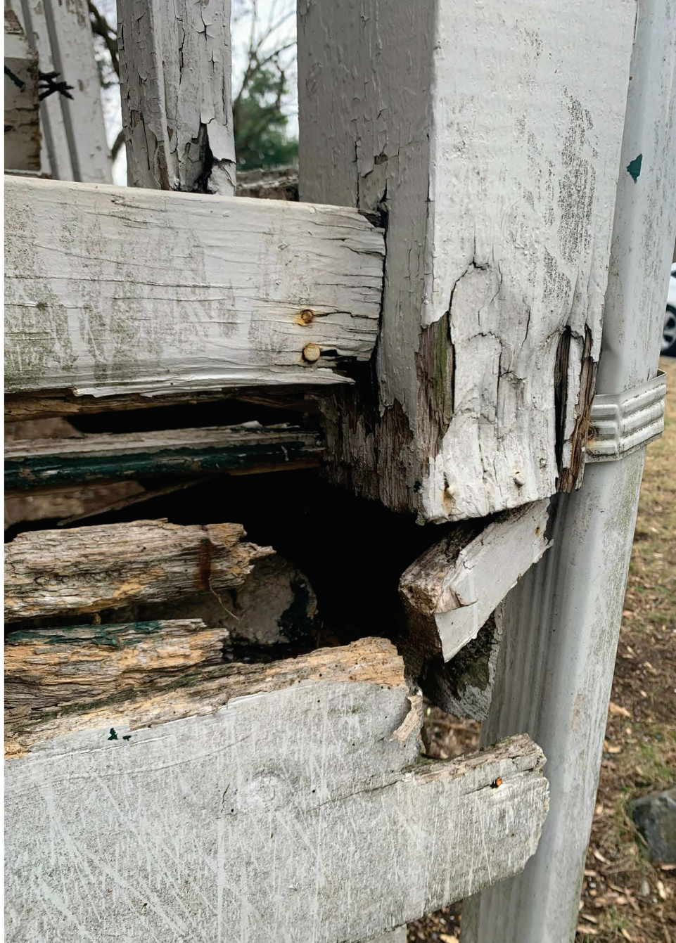
BMH Parsonage Decking, Railing and Post Condition- March 2026
