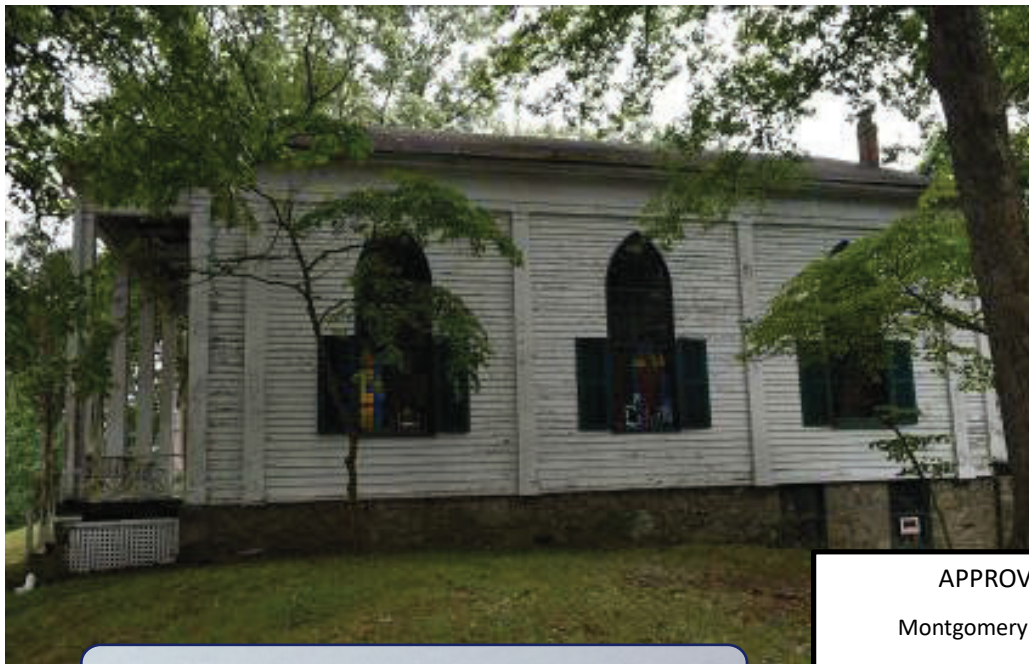
Bethesda Meeting House North Elevation View May 2025 By Laura DiPasquale at 9:31 am, May 14, 2026
