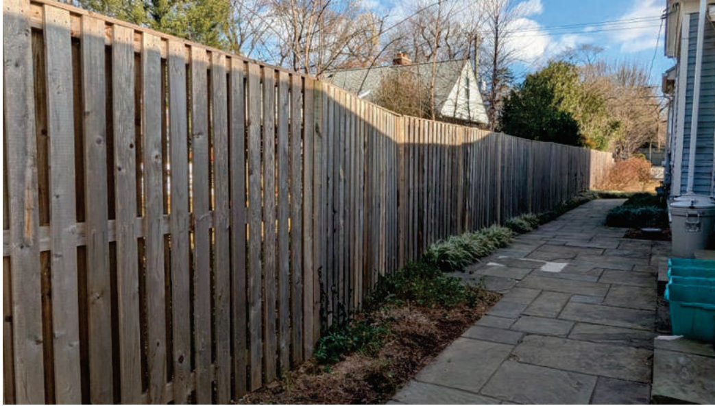
EXISTING: Existing “shadow-box fence along northern property line
