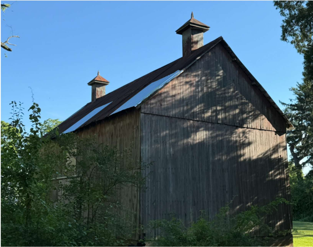
Figure 5. Rear (north) elevation. Faces neighbors / woods.
