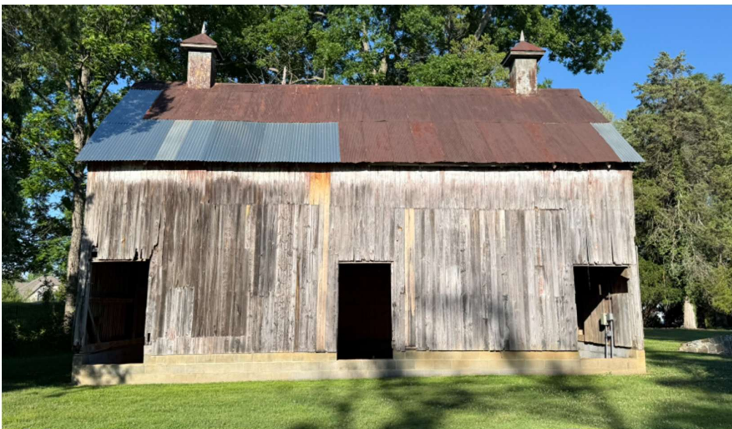
Figure 2. Side (west) Elevation facing stone cottage. Note roof panels that were replaced during prior repairs.
