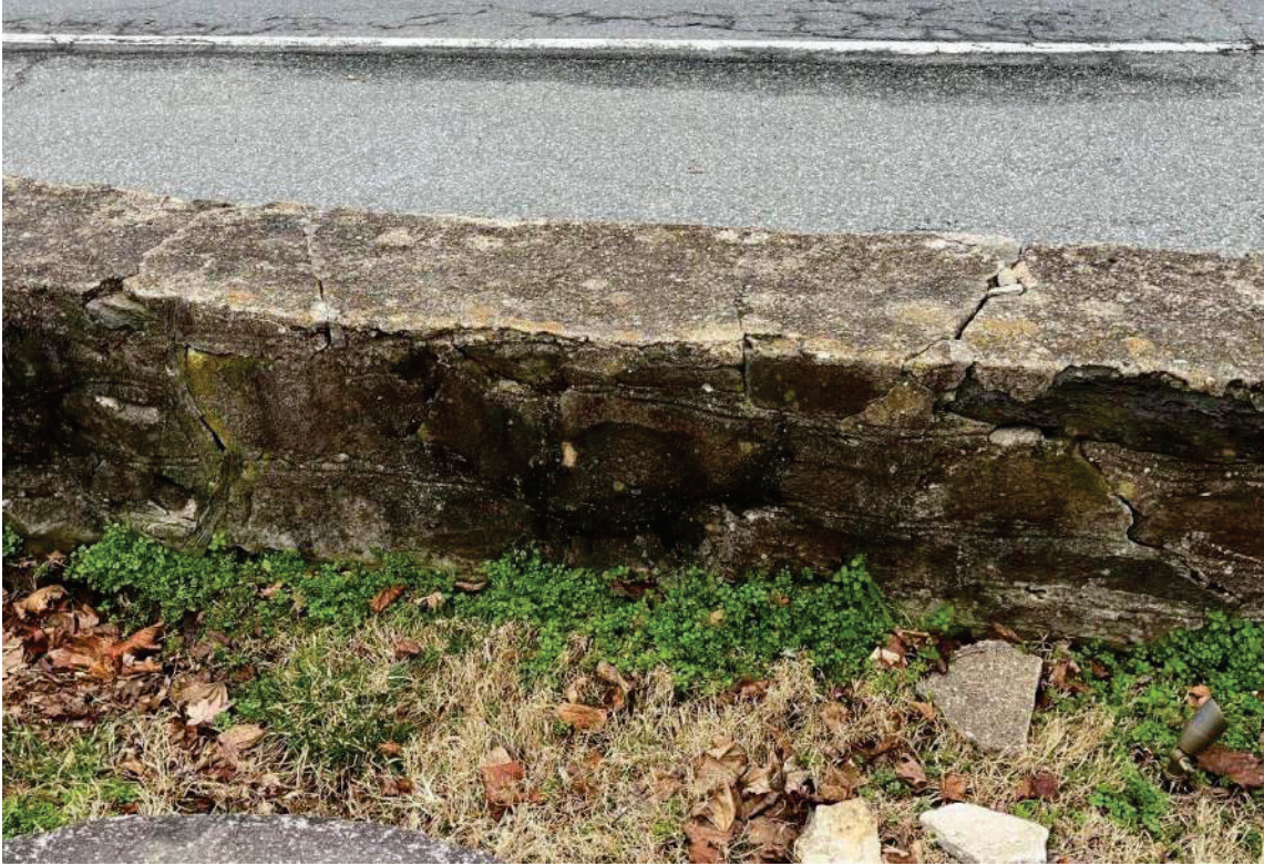
Photo 34 - Site Wall Close-Up 6
