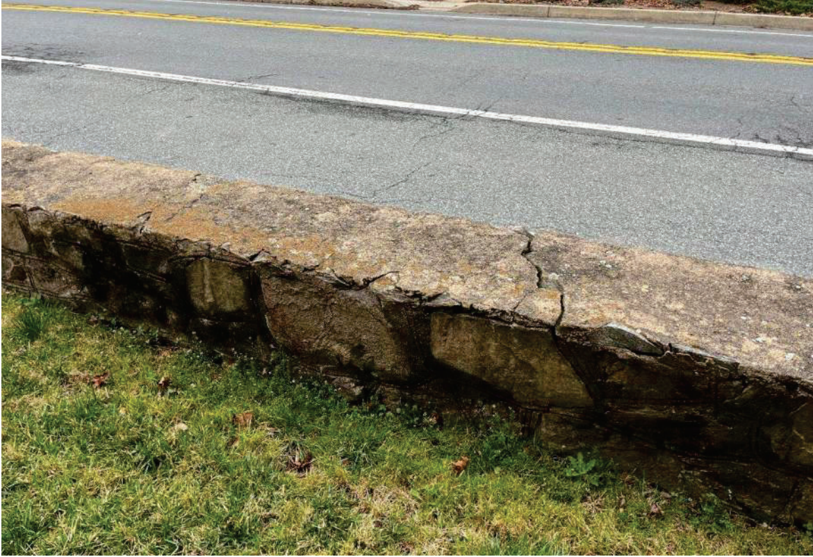
Photo 38 - Site Wall Close-Up 10
