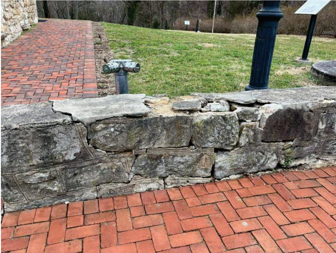
Photo 30 - Site Wall Close-Up 2
