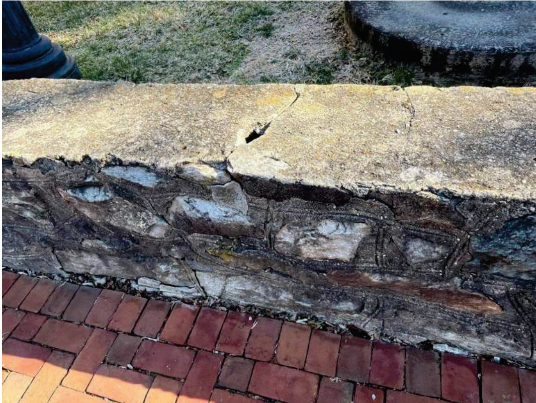
Photo 36 - Site Wall Close-Up 8
