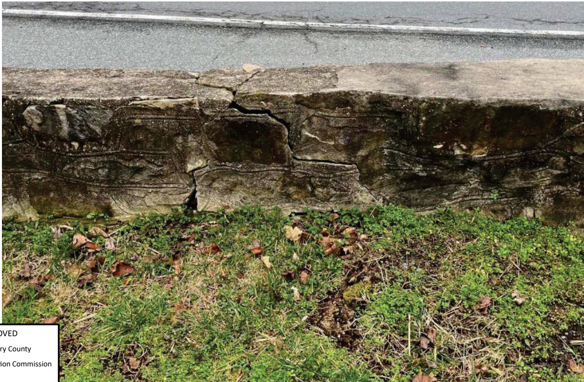
Photo 39 - Site Wall Close-Up 11
