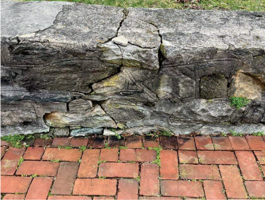
Photo 32 - Site Wall Close-Up 4
