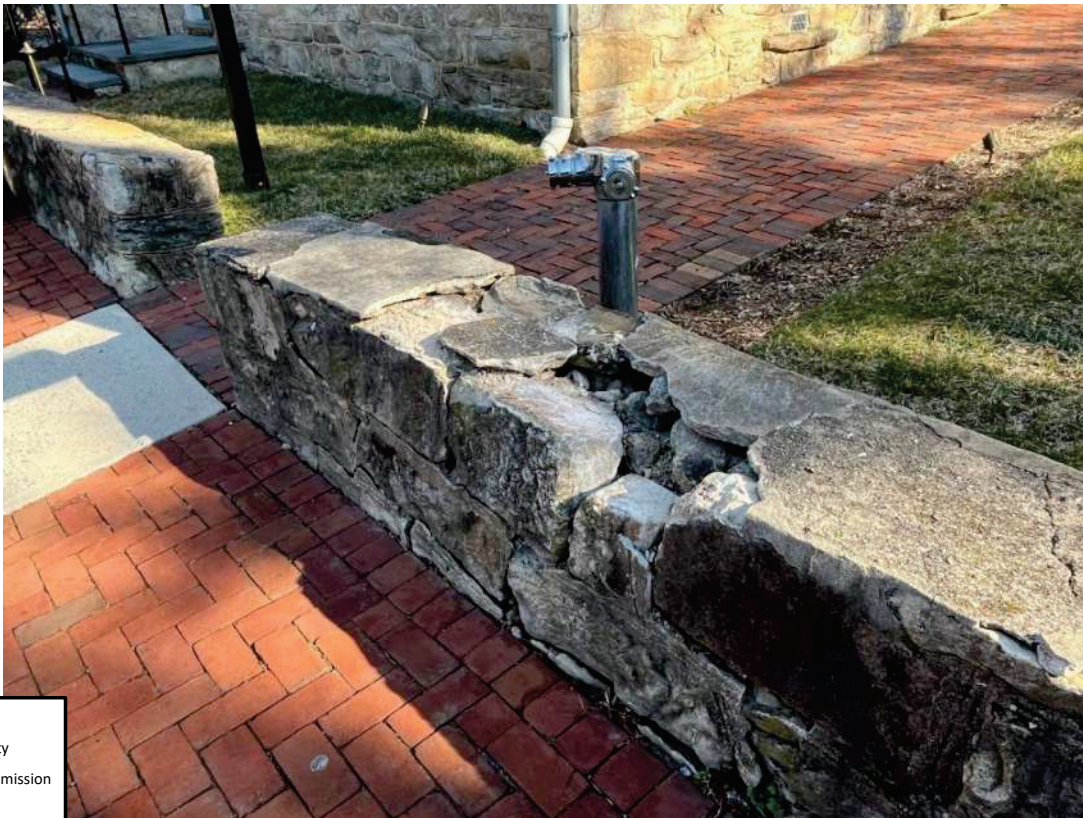
Photo 29 - Site Wall Close-Up 1
