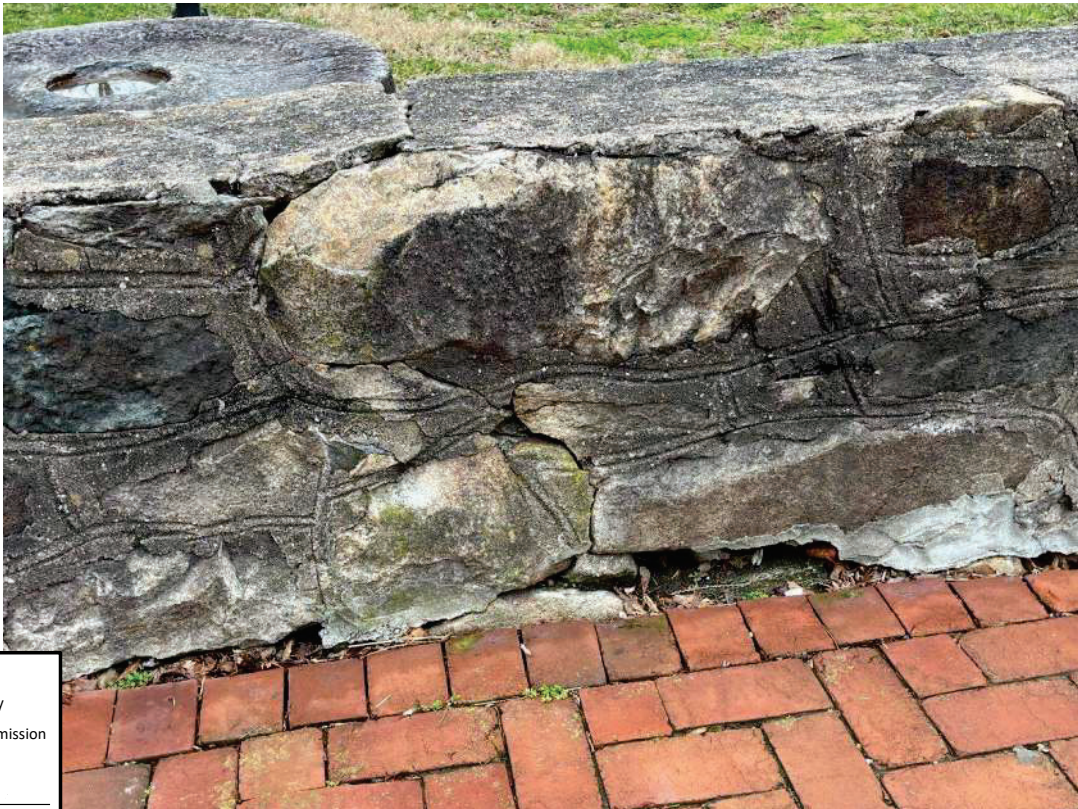
Photo 33 - Site Wall Close-Up 5
