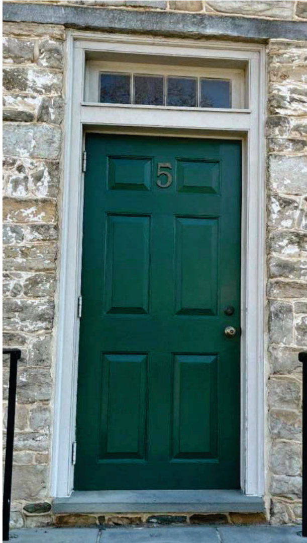
Photo 9 - Front Door Exterior
