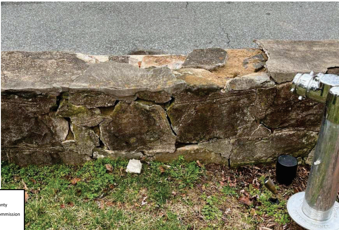
Photo 31 - Site Wall Close-Up 3
