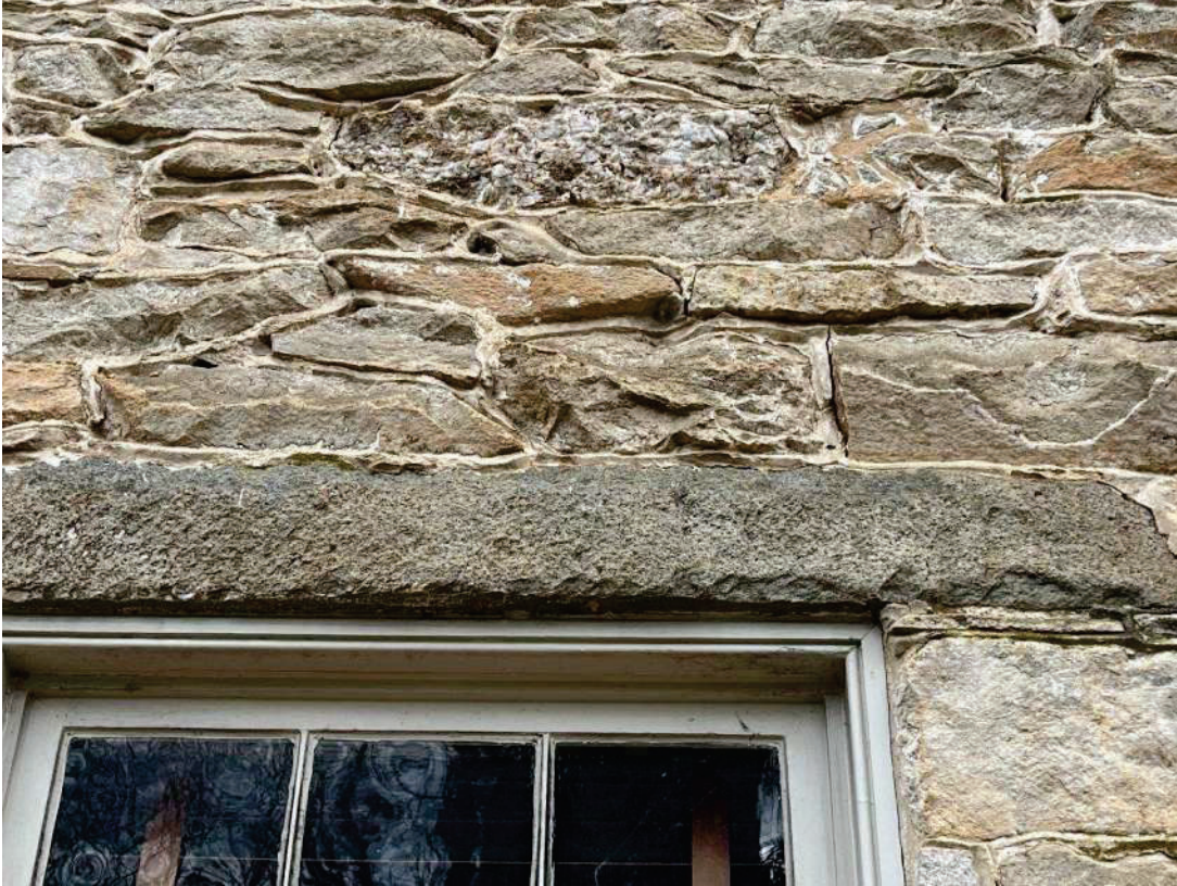
Photo 22 - Masonry Façade Close-Up 4
