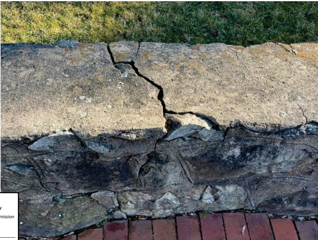
Photo 37 - Site Wall Close-Up 9
