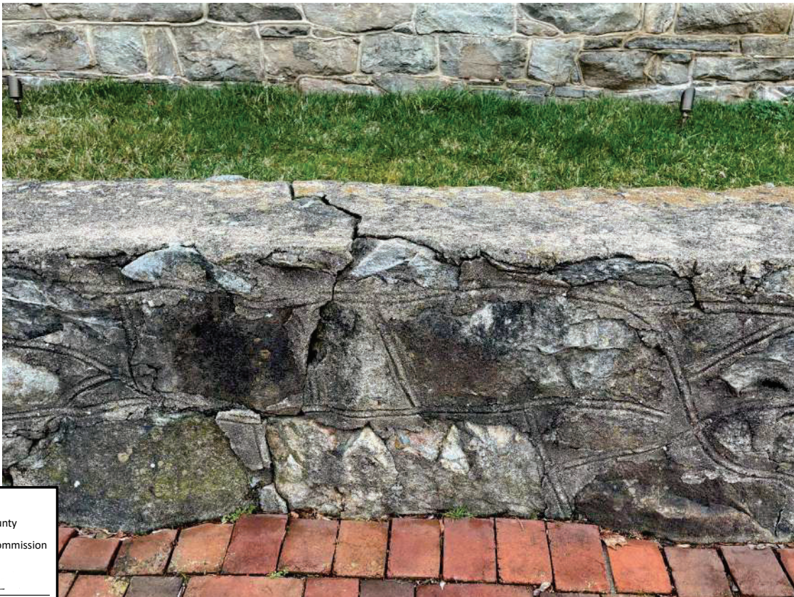
Photo 35 - Site Wall Close-Up 7
