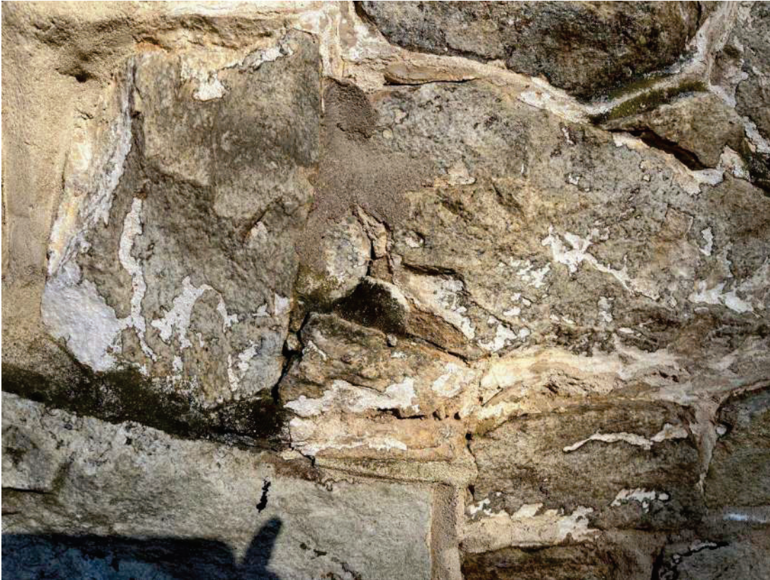
Photo 20 - Masonry Façade Close-Up 2
