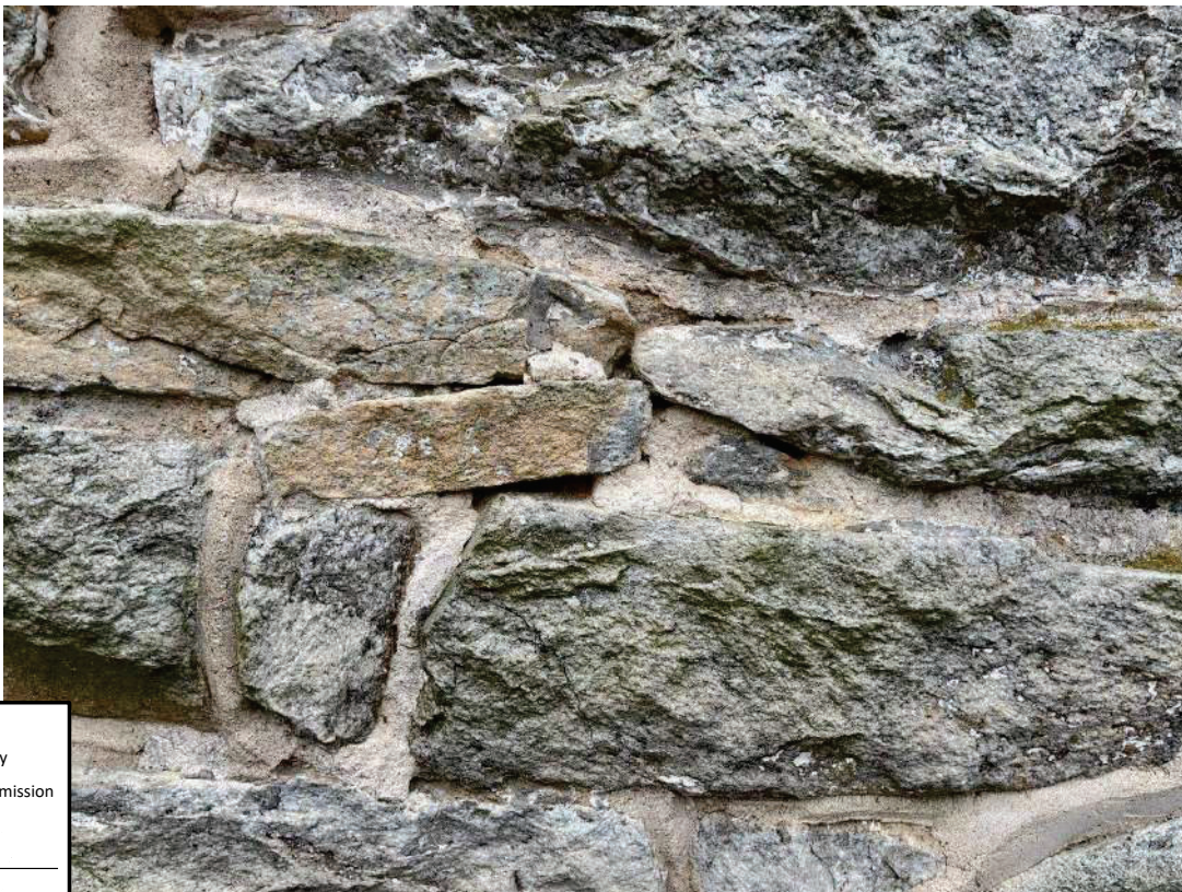
Photo 21 - Masonry Façade Close-Up 3
