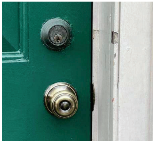
Photo 10 - Front Door Hardware Close-Up
