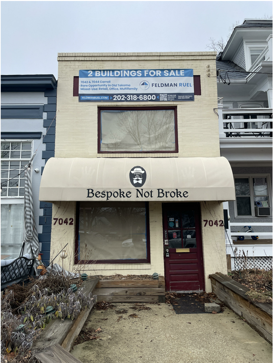
PHOTOGRAPH - EXISTING STOREFRONT
