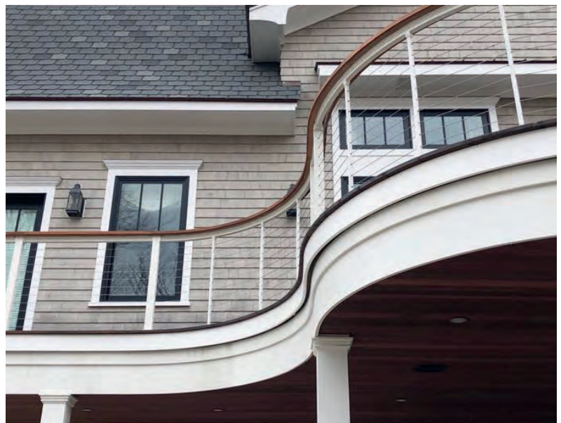
Courtesy of Sweenor Builders
