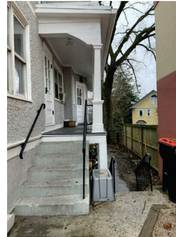
SIDE YARD ENTRY STAIR
