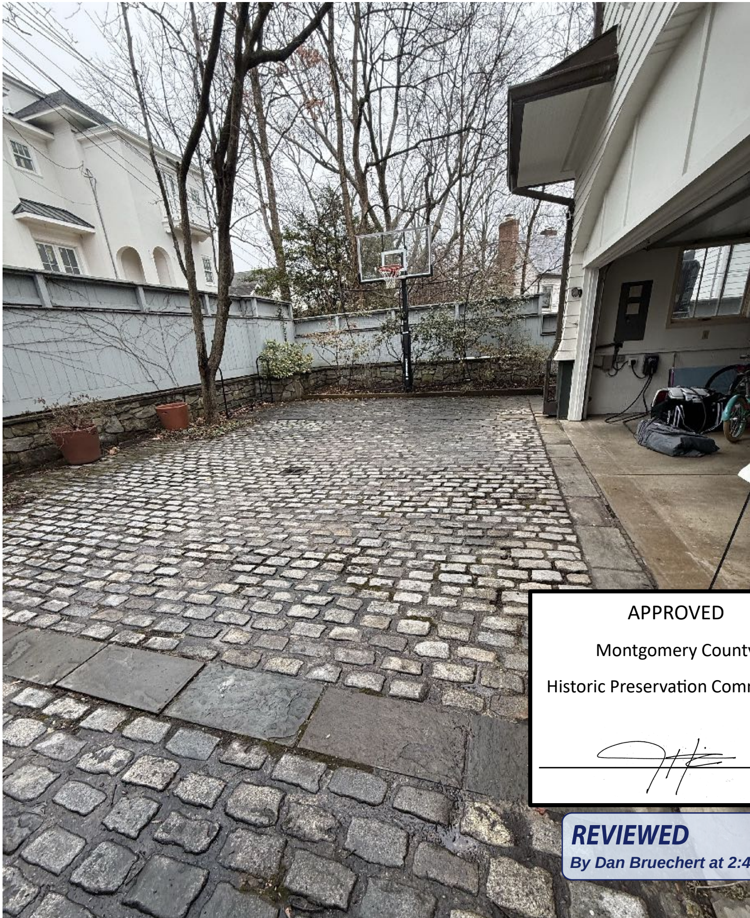
1 EXISTING COBBLESTONE DRIVEWAY. TO BE REPLACED WITH TAR AND CHIP OR CONCRETE AGGREGATE
