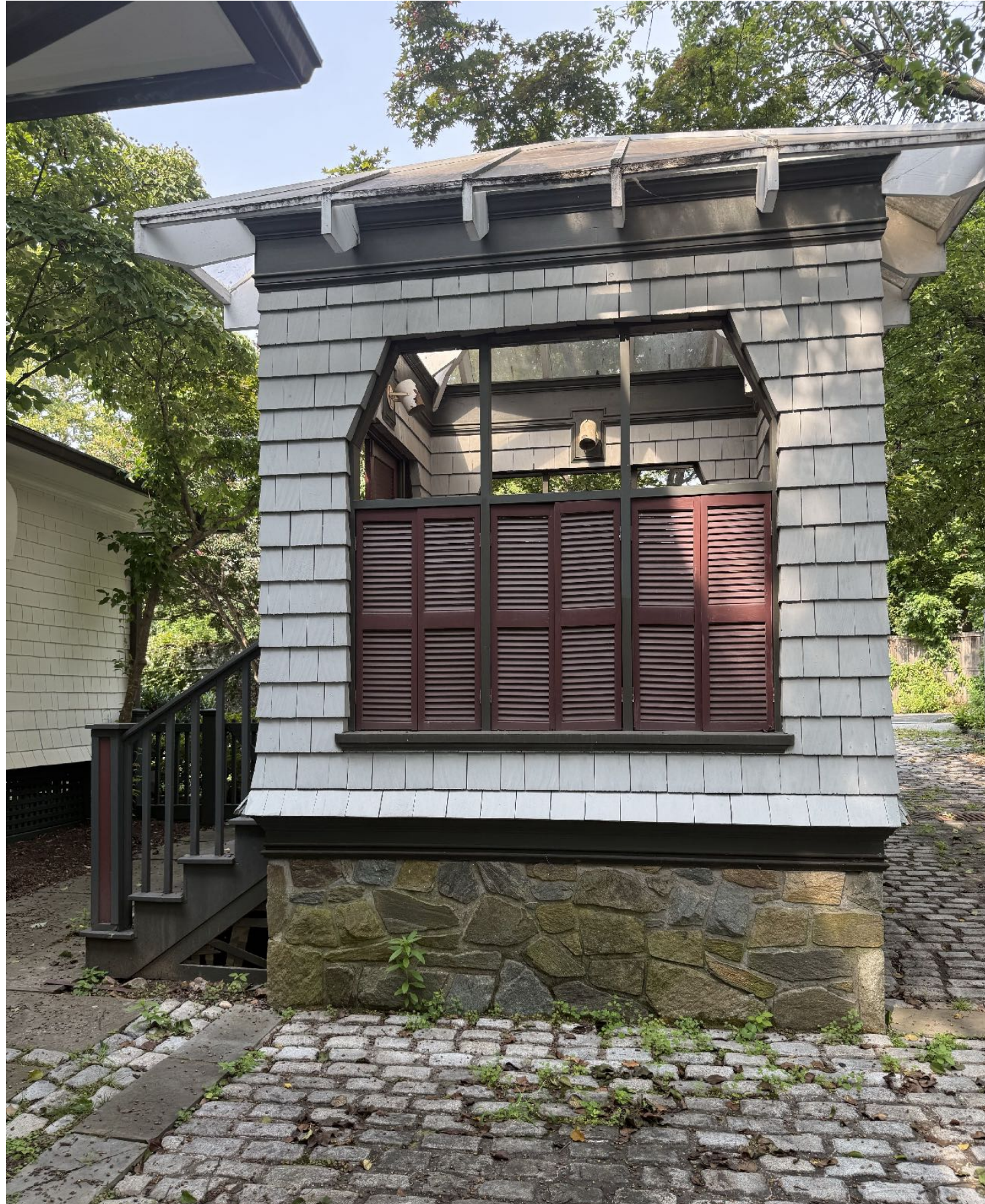
2 EXISTING GAZEBO STRUCTURE, TO BE REMOVED
