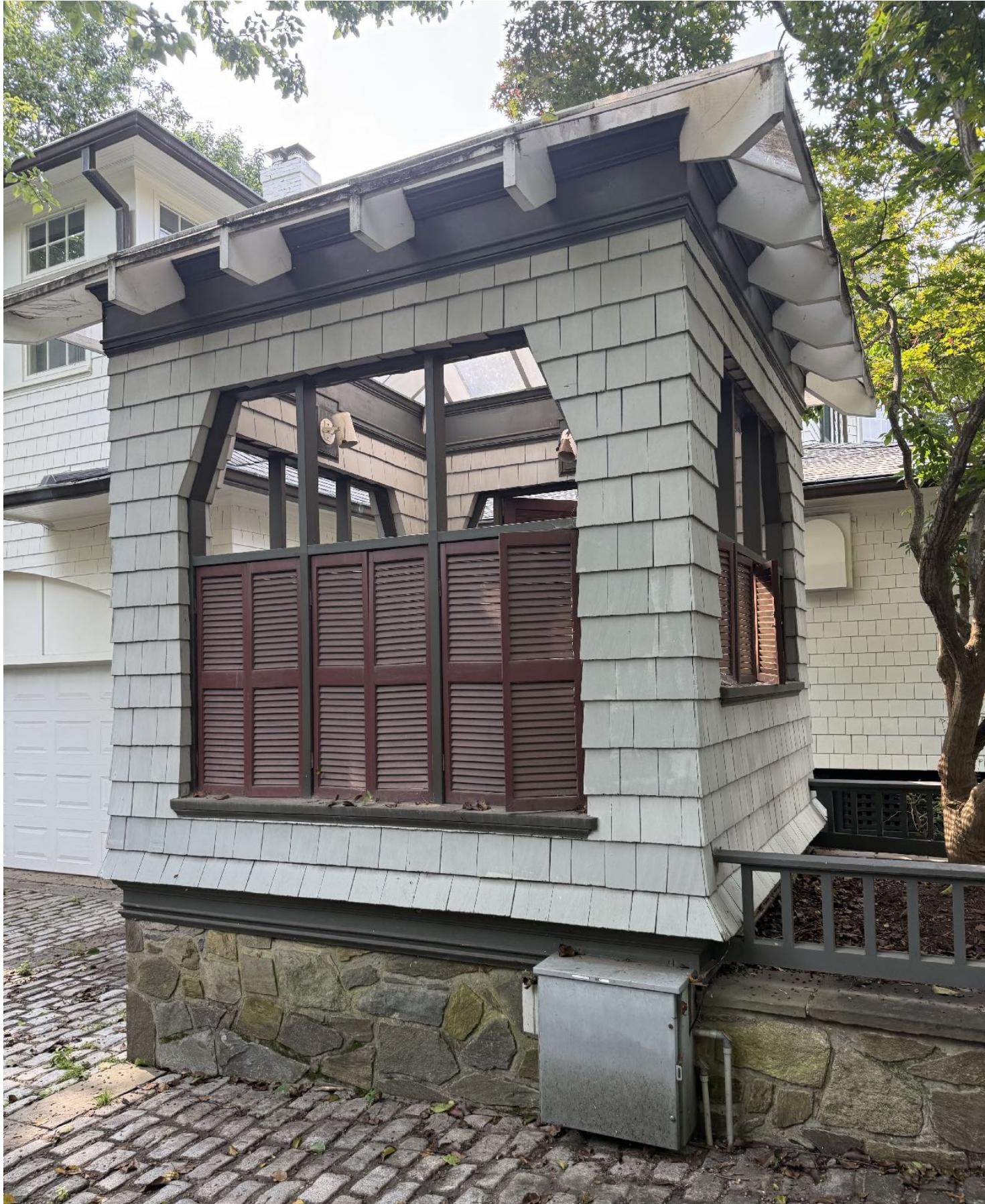
1 EXISTING GAZEBO STRUCTURE TO BE REMOVED
