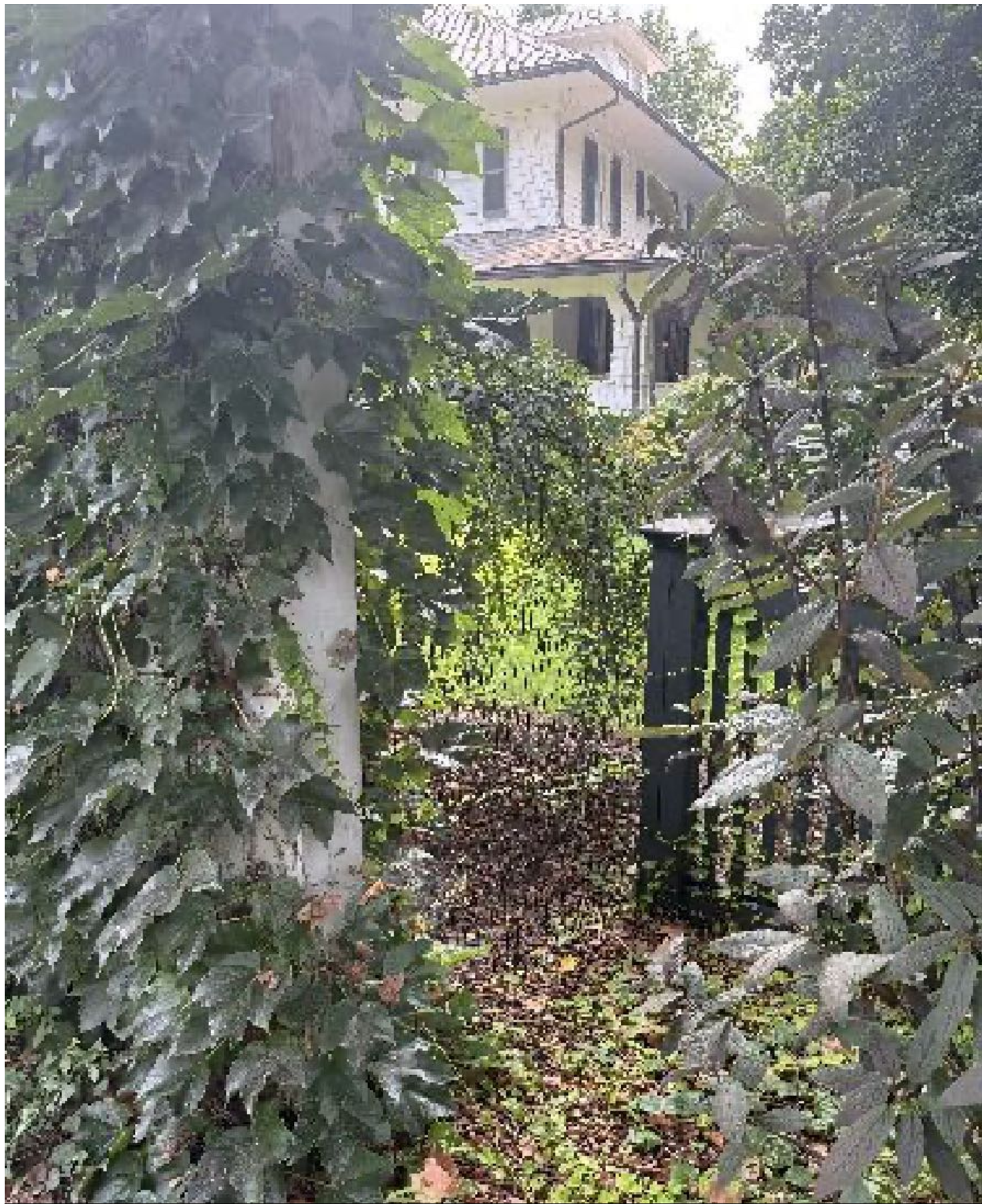
5 EXISTING SW CORNER FENCING. WIRE CHICKEN FENCE TO BE REMOVED AND REPLACED WITH WOOD PICKET FENCING, TO MATCH EXISTING.
