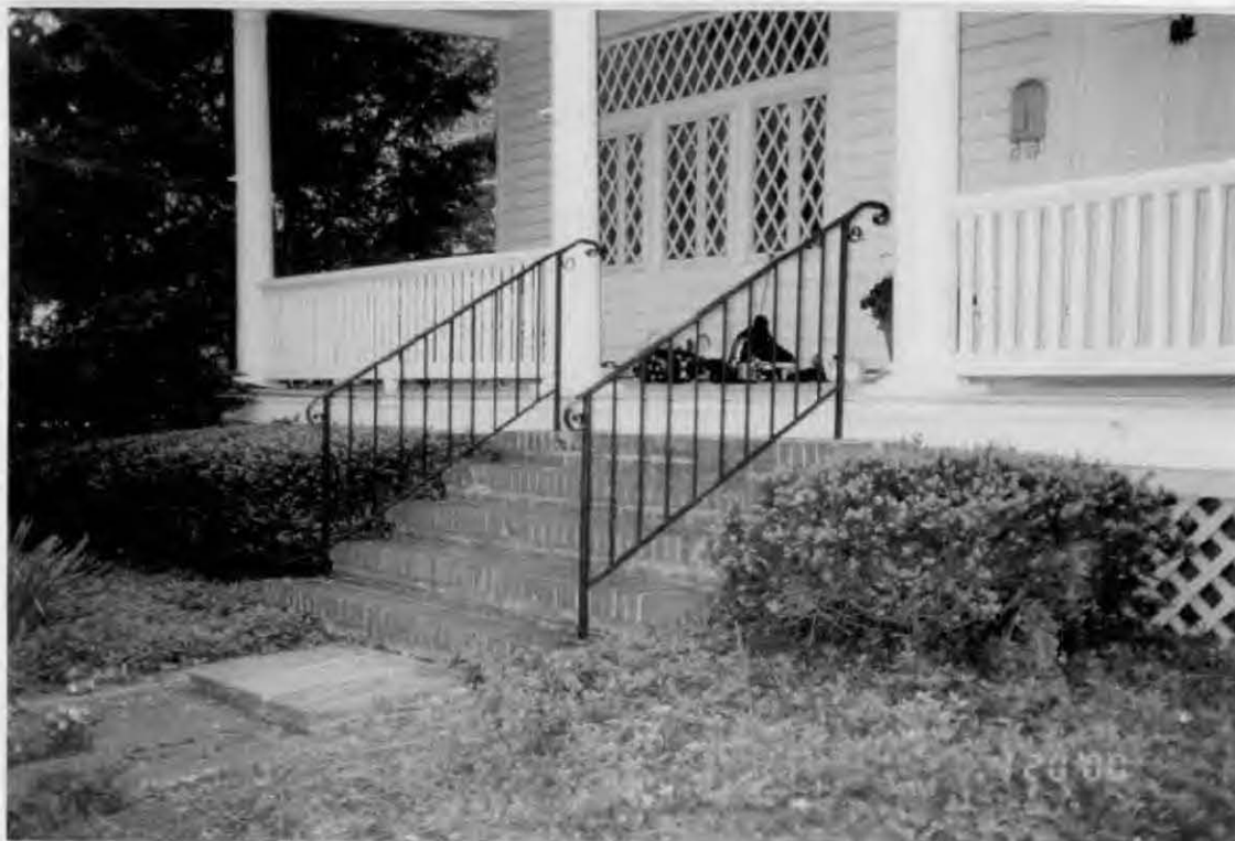
Close up of existing steps - #7 East Melrose
