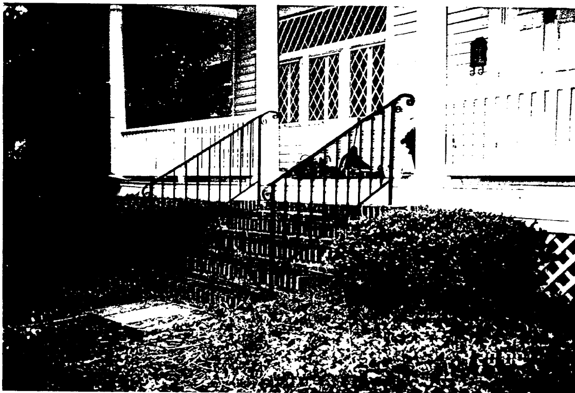
Close up of existing steps - #7 East Melrose
