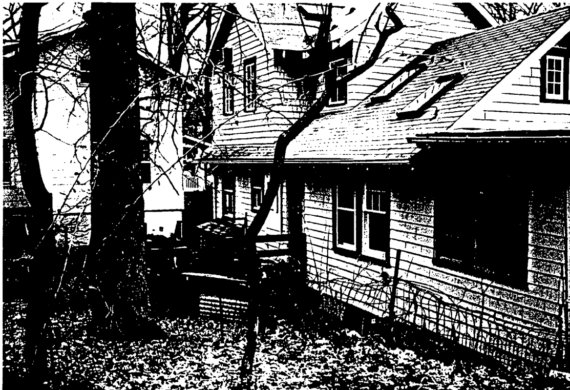
Photo 7: View of the rear of the house. The new roof structure will not adversely affect the look of the house from the rear.
