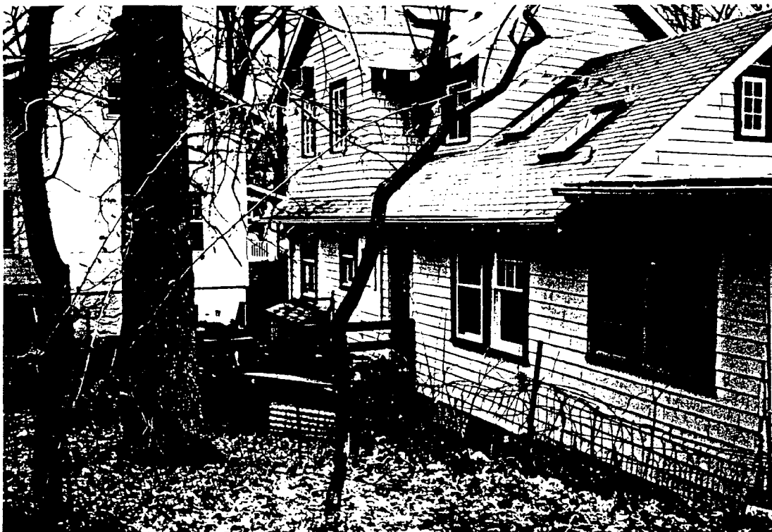
Photo 7: View of the rear of the house. The new roof structure will not adversely affect the look of the house from the rear.
