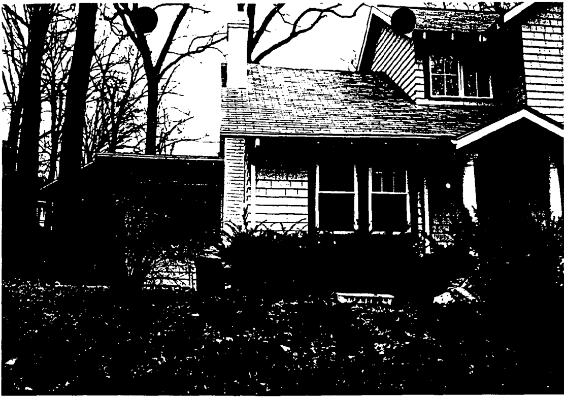
Photo 4: View of the front of the existing addition, as seen from the street. Due to the difference in elevation, it is not possible to see the roof of the addition.
