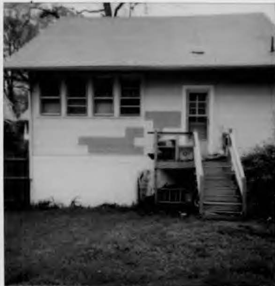
Existing porch 7210 Spruce Ave TP Md.
