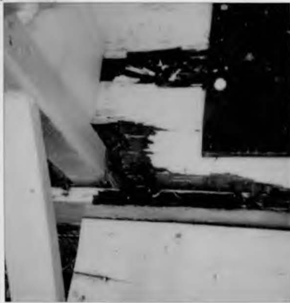
Existing porch 7210 Spruce Ave TP Md
