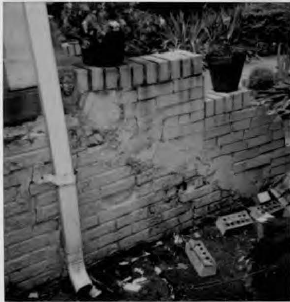
SOUTH SIDE OF FRONT PORCH STEPS
