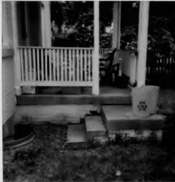
REAR NW CORNER PROPOSED DECK LOCATION 9 PINE AVE.
