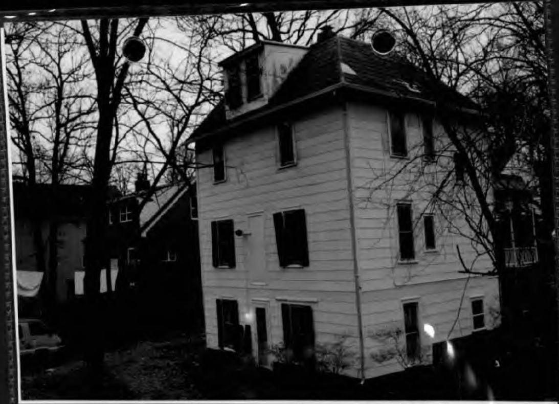
View from North East
