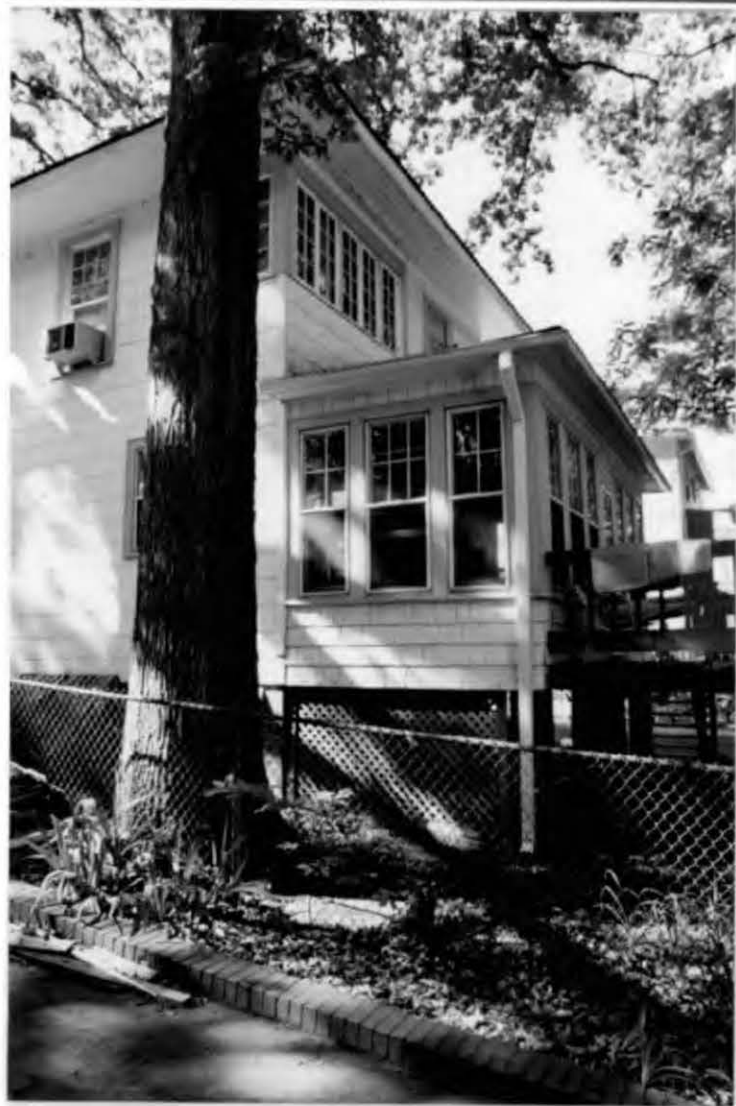
EXISTING REAR STRUCTURE
