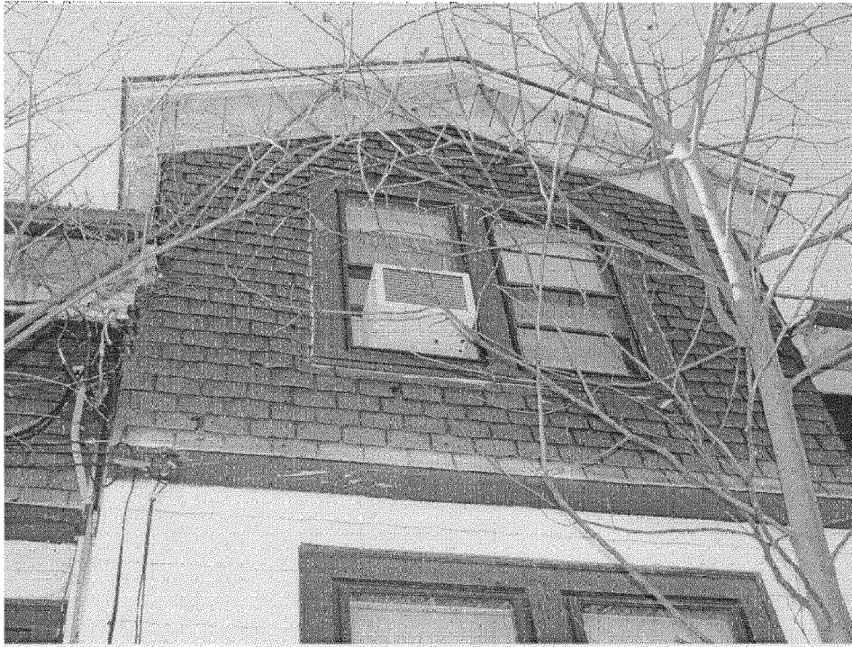
Asphalt shingling on upper wall surface
