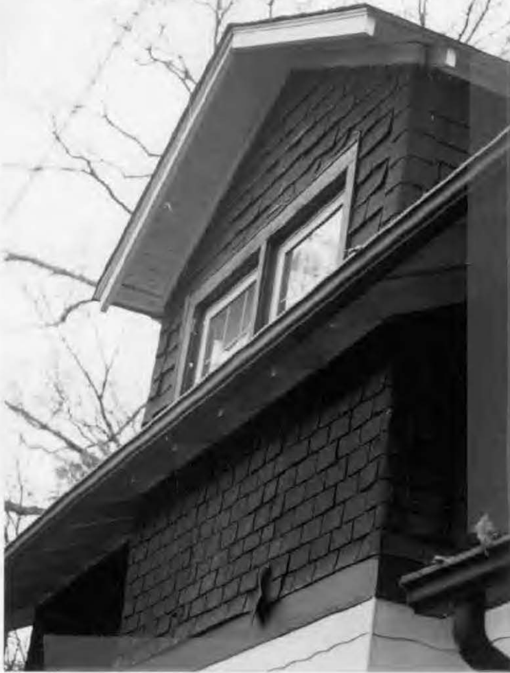
Condition of 2nd floor shingles.
