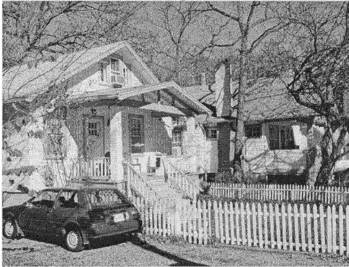
Two houses to the east – asbestos shingling
