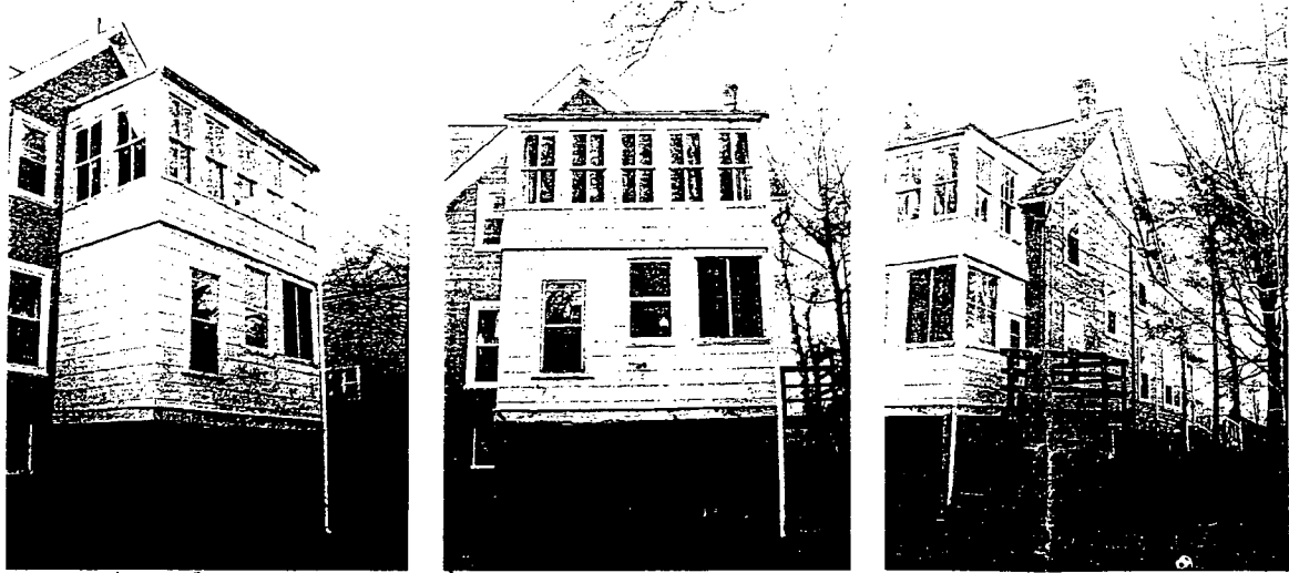
EXISTING REAR ADDITION
