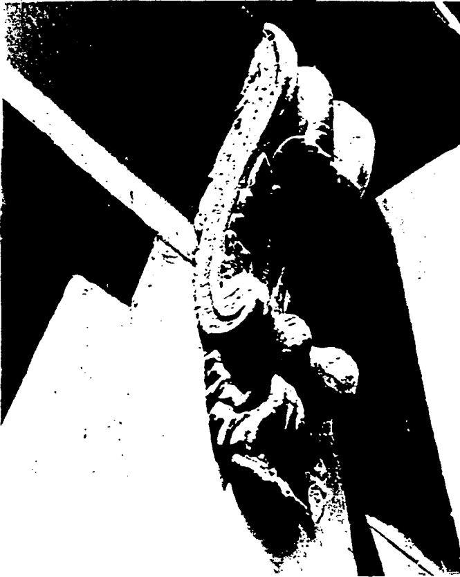
Fig. 1 Excessive paint build-up on architectural details such as this ornamental bracket does not in itself justify total paint removal. If paint is cracked and peeling down to bare wood, however, it should be removed using the gentlest means possible. Photo: David W. Look, AIA.
