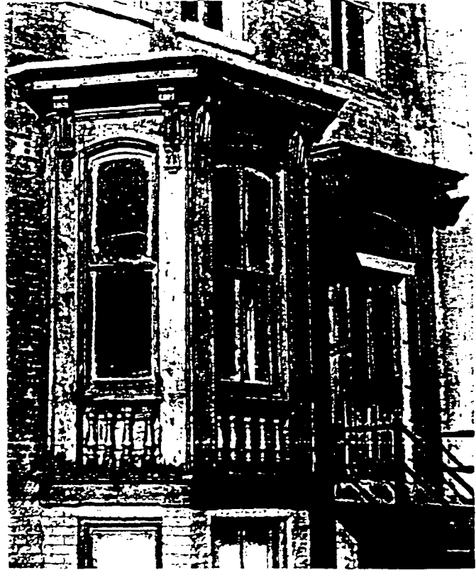
Fig. 2 A traditionally painted bay window has been stripped to bare wood, then painted in an attempt to being historically inaccurate. The finish will break down faster as a result of the sun's ultraviolet rays than would primer and finish coats of paint. Photo: David W. Look. AIA.
