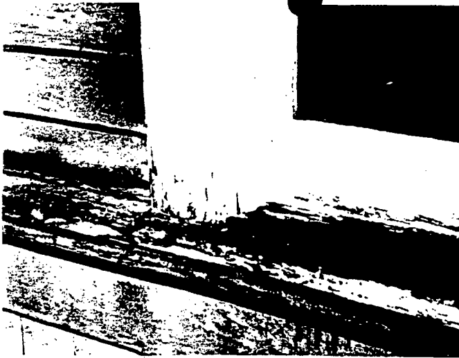
Figure 3. Deterioration of poorly maintained windows usually begins on horizontal surfaces and at joints where water can collect and saturate the wood. The problem areas are clearly indicated by paint failure due to moisture. Photo: Baird M. Smith, AIA
