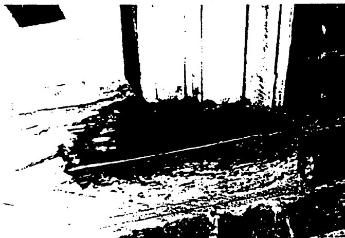
Figure 5. This illustrates a two-part epoxy patching compound used to fill the surface of a weathered sill and rebuild the missing edge. When the epoxy cures, it can be sanded smooth and painted to achieve a durable and waterproof repair. Photo: John H. Myers
