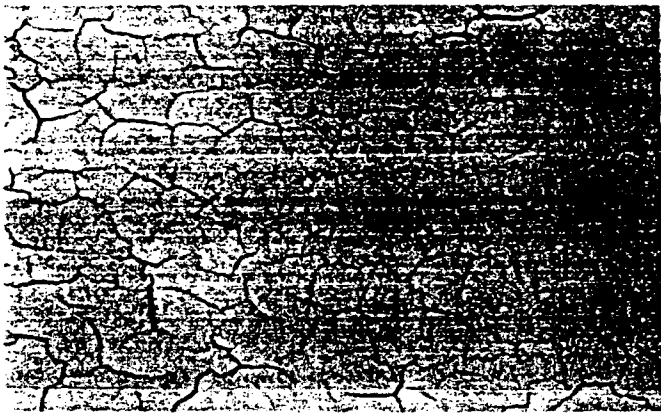
Fig. 5 Crazing—or surface cracking—is an exterior surface condition which can be successfully treated by sanding and painting. Photo: Courtesy, National Decorating Products Association.
