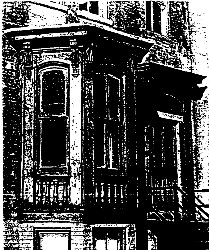
Fig. 2 A traditionally painted bay window has been stripped to bare wood, then varnished. In addition to being historically inaccurate, the varnish will break down faster as a result of the sun's ultraviolet rays than would primer and finish coats of paint. Photo: David W. Look, AIA.
