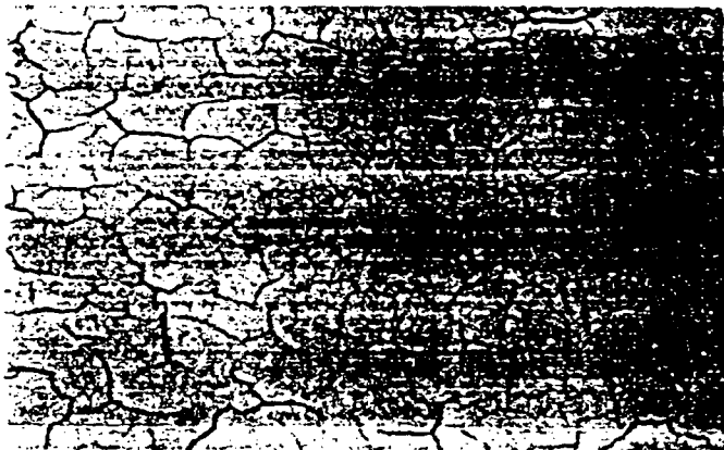
Fig. 5 Crazing—or surface cracking—is an exterior surface condition which can be successfully treated by sanding and painting. Photo: Courtesy, National Decorating Products Association.
