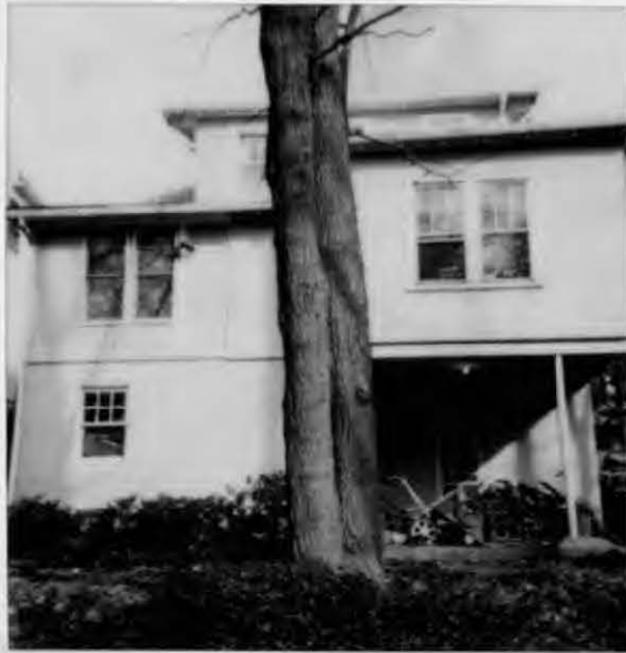
Patch - 7112 Sycamore Ave TP rear view
