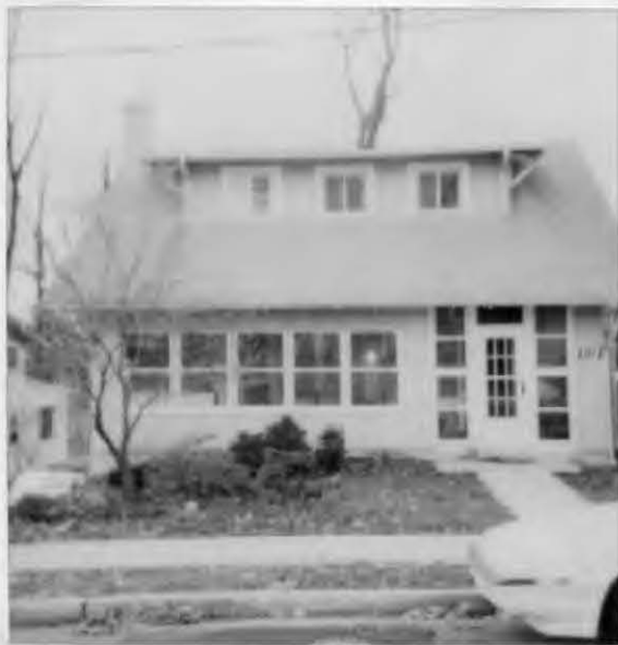
Patch, 7112 Sycamore Ave, TP front view
