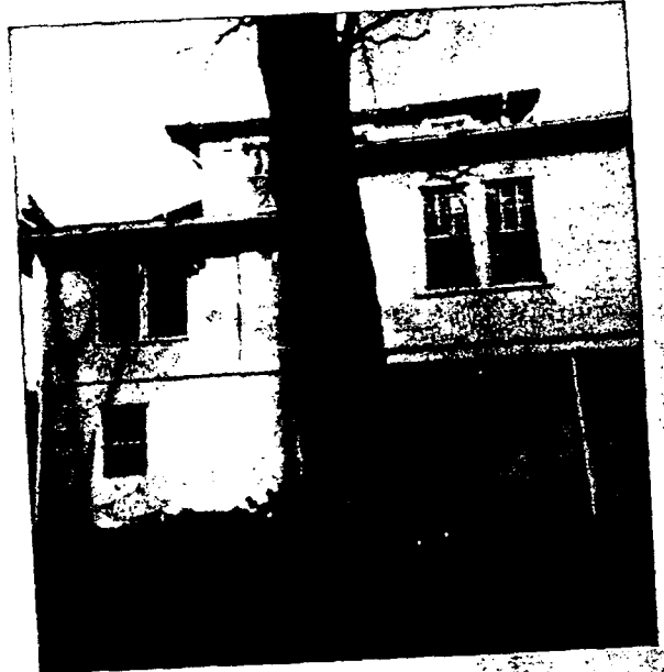
Patch - 7112 Sycamore Ave TP rear view
