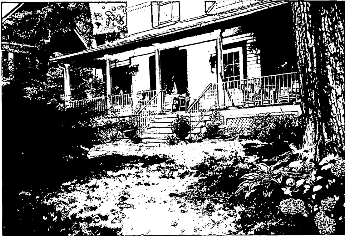
Metal Railing at Front Porch
