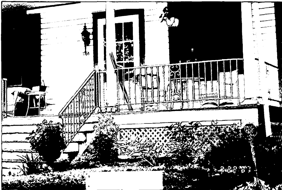
CLOSE-UP VIEW OF METAL RAILING
