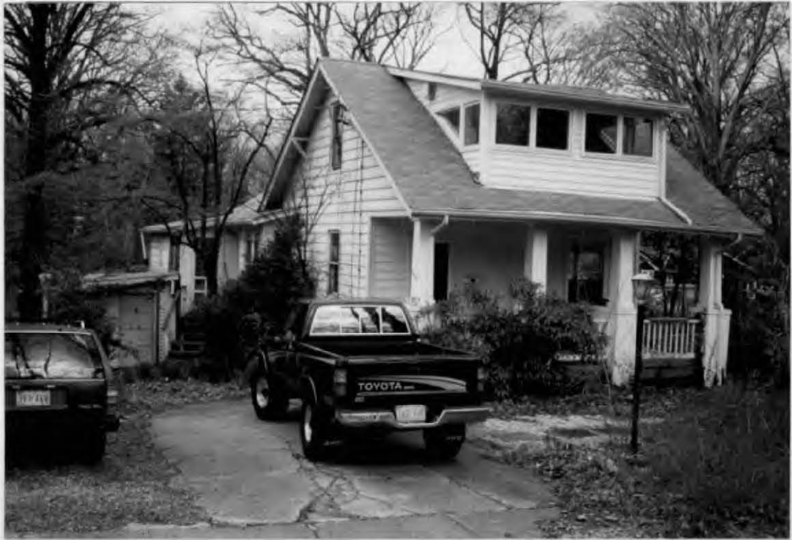
FRONT OF SUBJECT BUILDING
