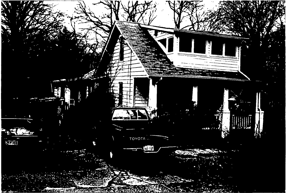
FRONT OF SUBJECT BUILDING
