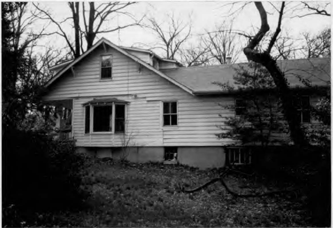
SIDE OF SUBJECT BUILDING SHOWING SIMILAR DORMER TO BE CONSTRUCTED
