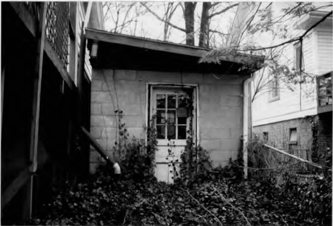
REAR OF SHED FACING EAST
