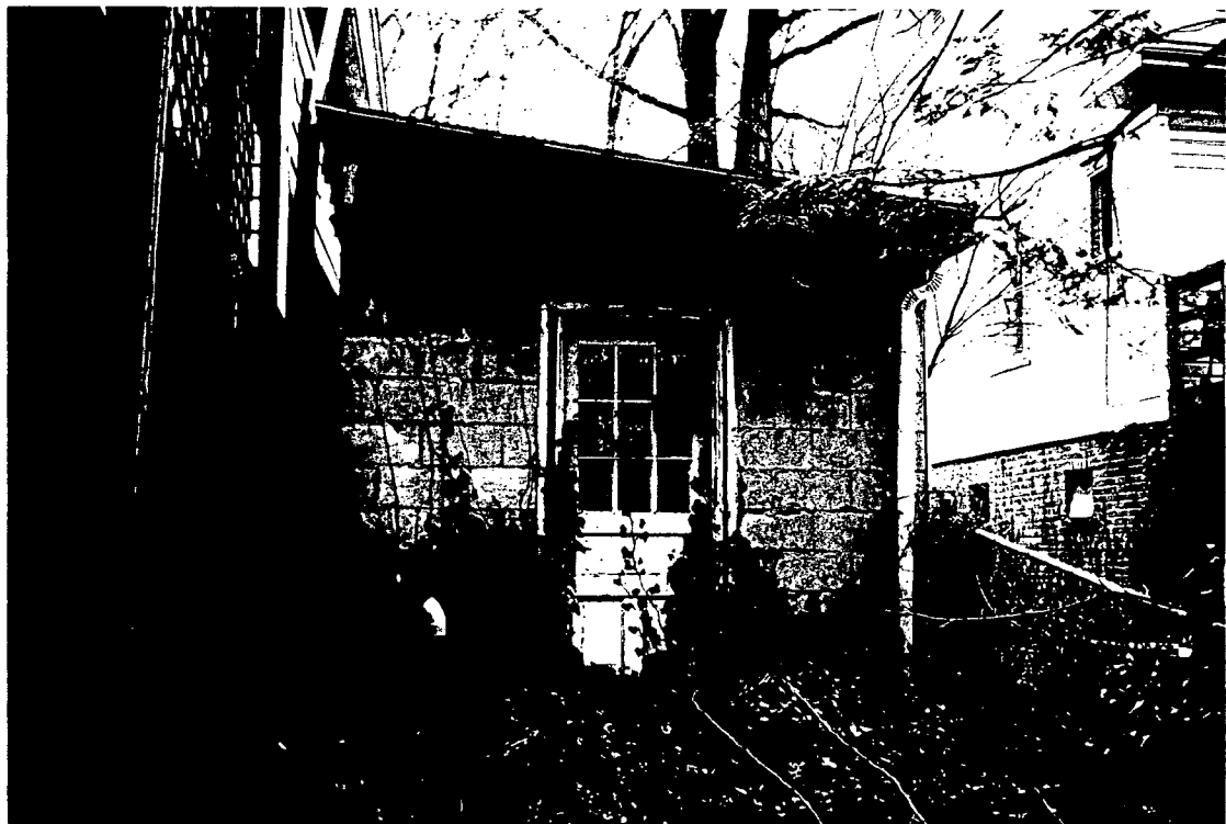
REAR OF SHED FACING EAST
