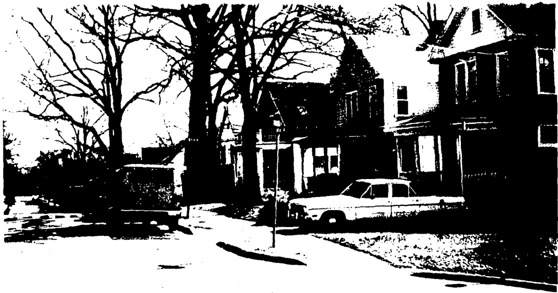
Looking South on Sycamore Ave
