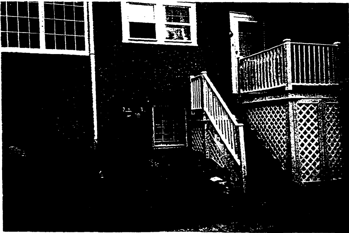
SIDE VIEW (NE) - CLOSE-UP
