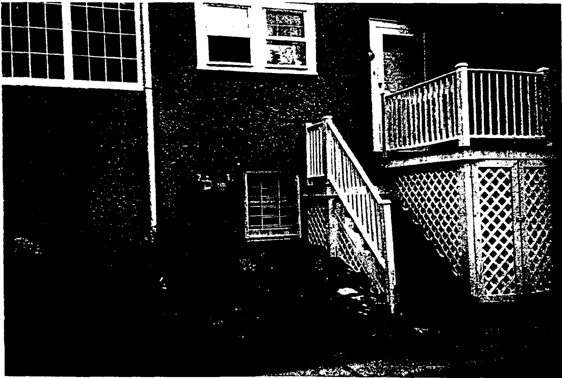
SIDE VIEW (NE) - CLOSE-UP
