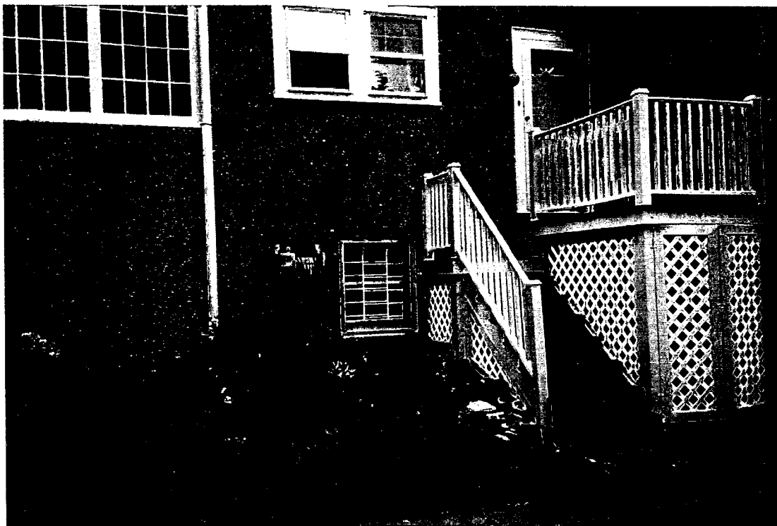
SIDE VIEW (NE) - CLOSE-UP
