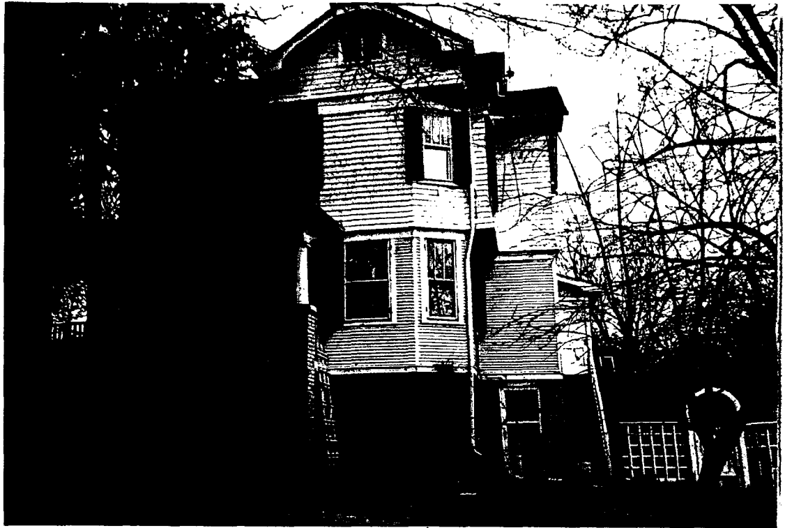
South (side) facade
