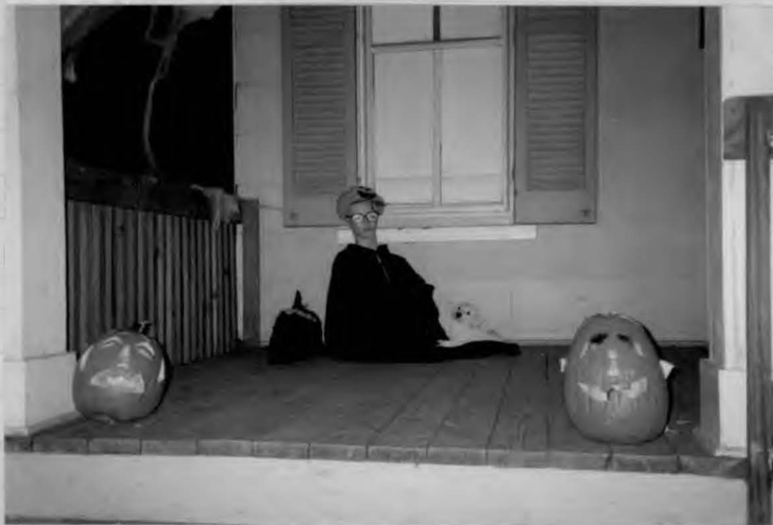
Shows ① Aluminum Storm window ② Wood Porch Flooring 2" x 6" ④ Front Stairs to Left
