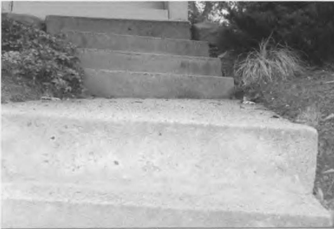
Photo 4: two lower steps settled to right; three upper steps slanted to right; top step (beginning of apron) straight and lowest porch step in view slanted to right.
