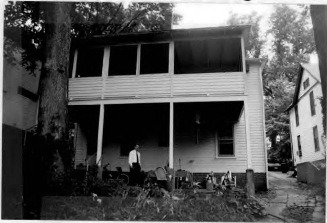
VIEW OF REAR ELEVATION
