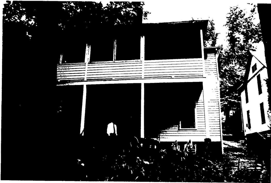
VIEW OF REAR ELEVATION
