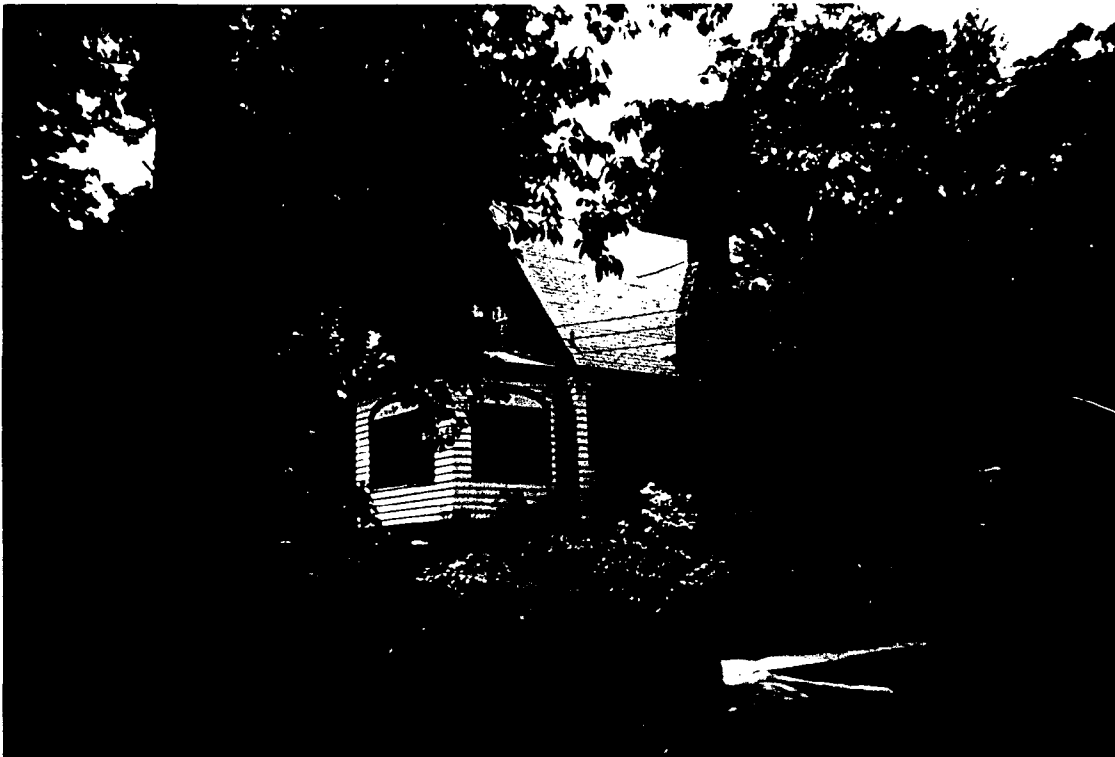
VIEW OF SIDE PORCH - LOCATION OF PROPOSED NEW ADDITION
