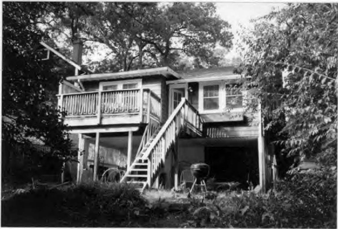
View from backyard - original house
