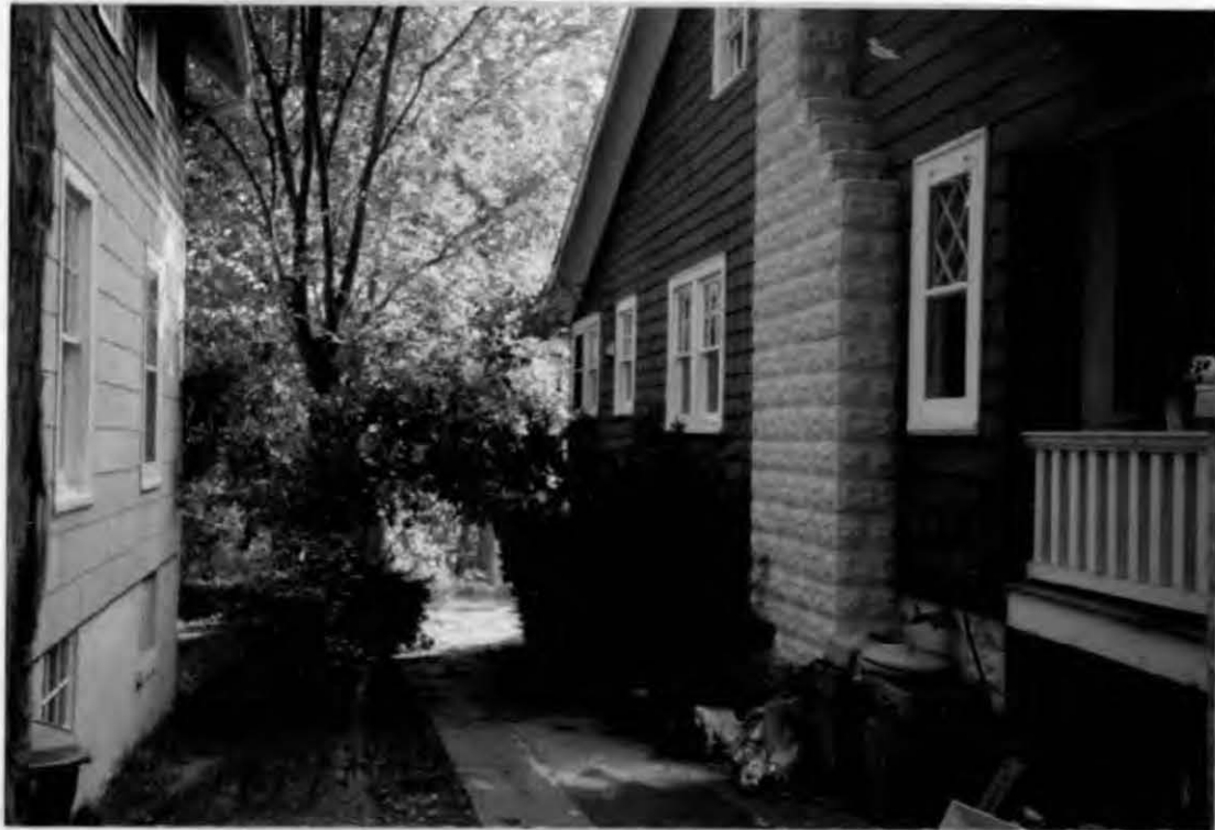
View from driveway
